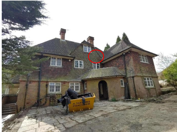
Photograph 1. North elevation of Hurstmead showing hanging tiles and location of bat roost circled in red.
