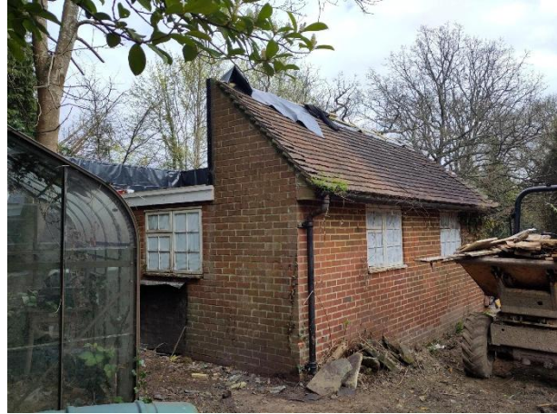
Photograph 10. Building B2 located to the northeast of B1 and not subject to emergence surveys.
