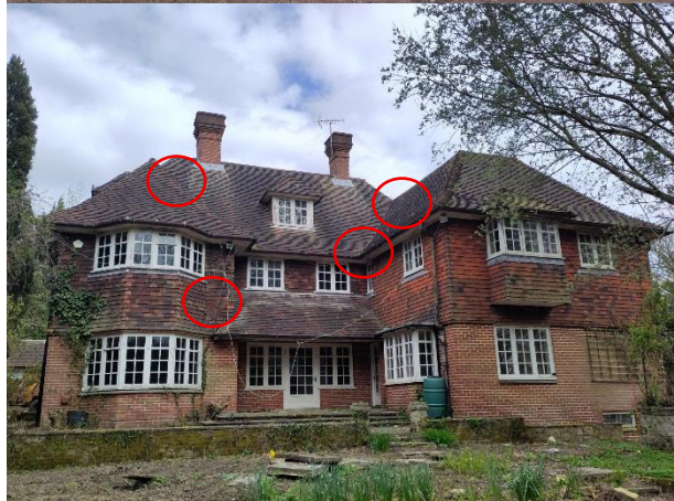
Photograph 3. South elevation of Hurstmead showing hanging tiles and location of bat roost circled in red.
