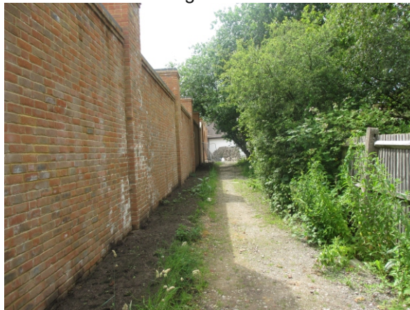
Photograph 3. View of the ground between the wall and fence looking SE
