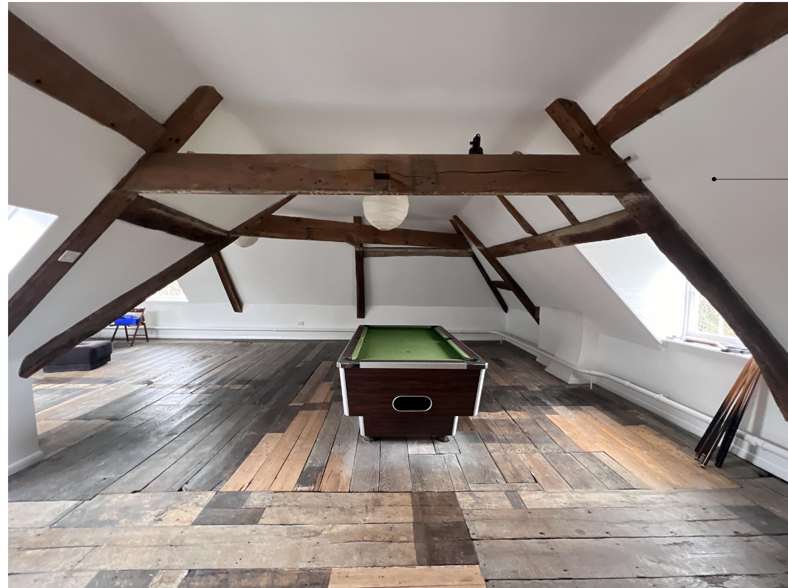
Sunte House - Roof Space
