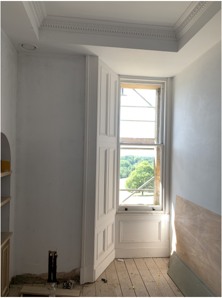
Image of non original wall and dropped ceiling.
