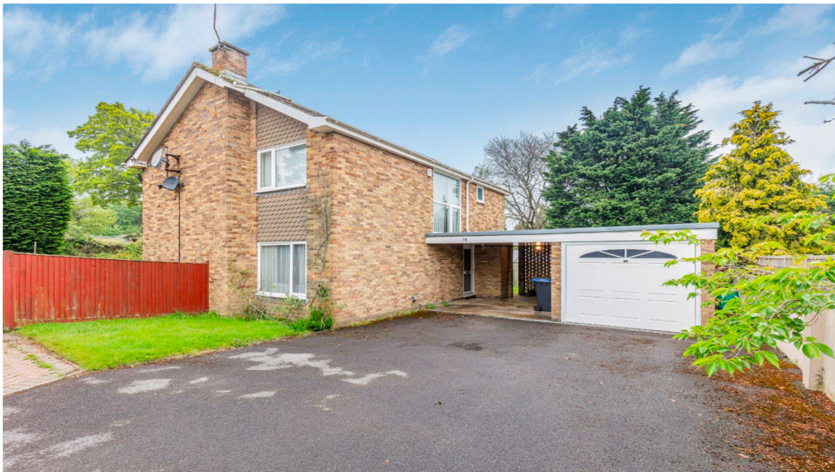
View looking north-west showing front & side elevation and garage/carport
