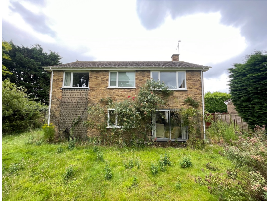
View looking north-east showing rear elevation
