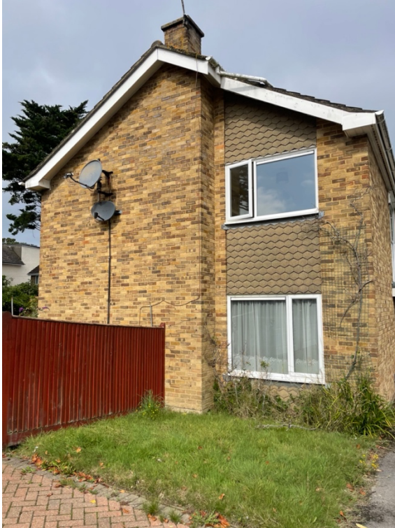
View looking north-west showing front elevation
