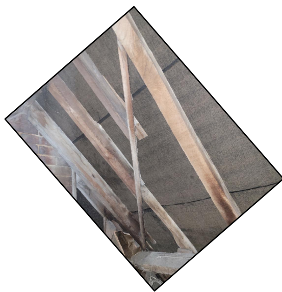
RAFTERS AT ROOFLIGHT 1
