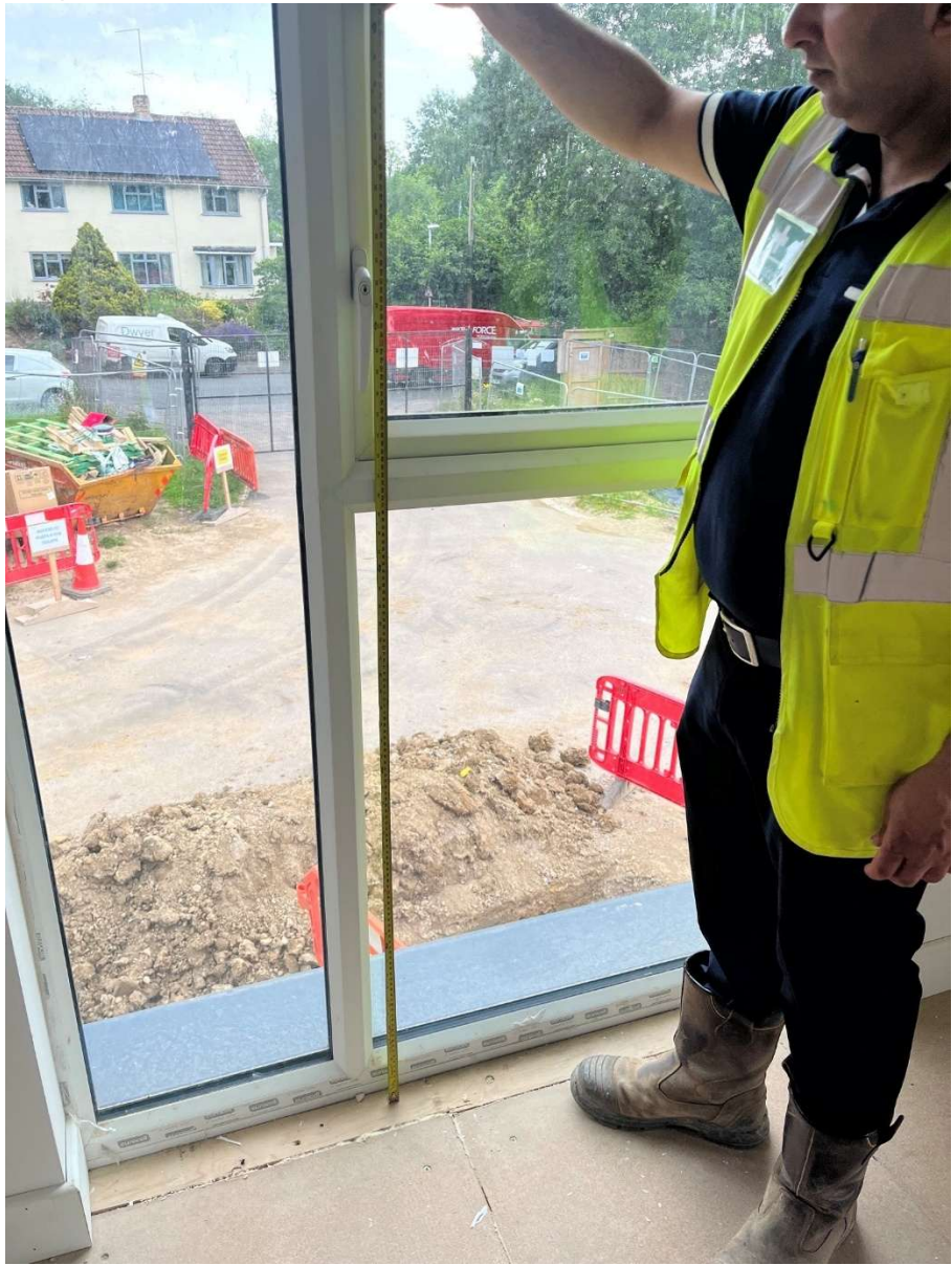
Plot 7's top of handles are 1300mm from FFL.
