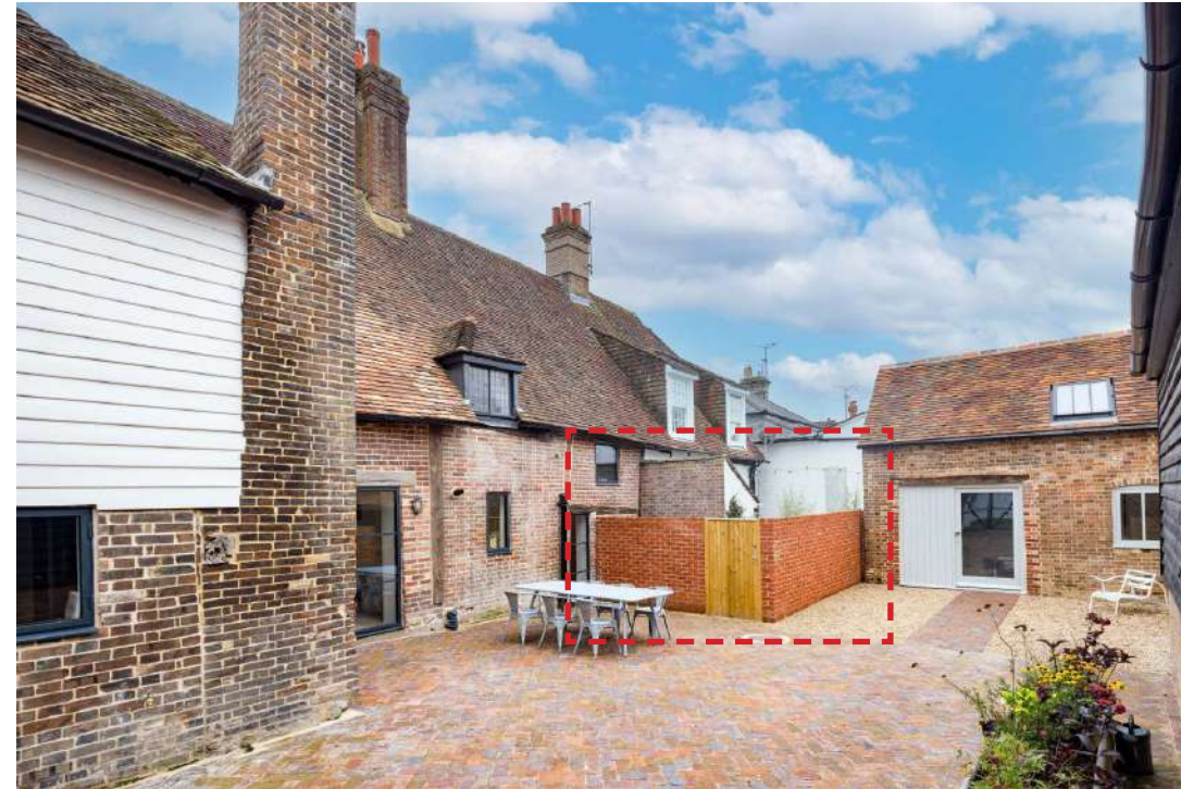
As-built rear brickwork wall
