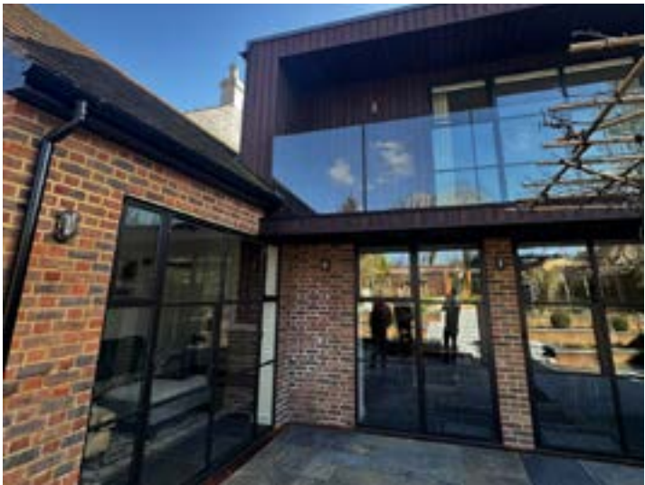
Rear elevation & re-constructed bake house
