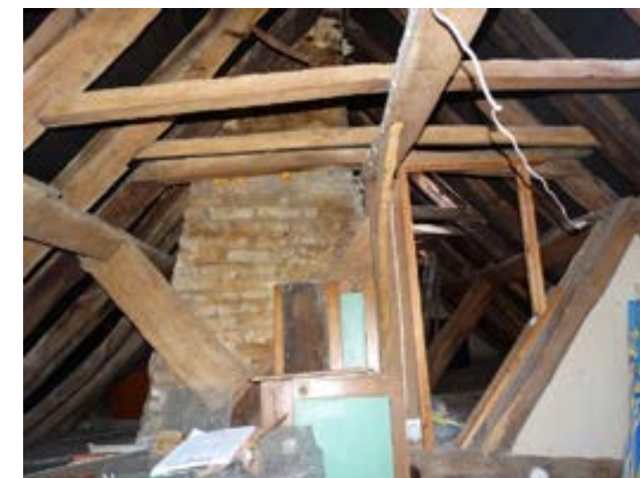
Attic, chimney stack in the background
