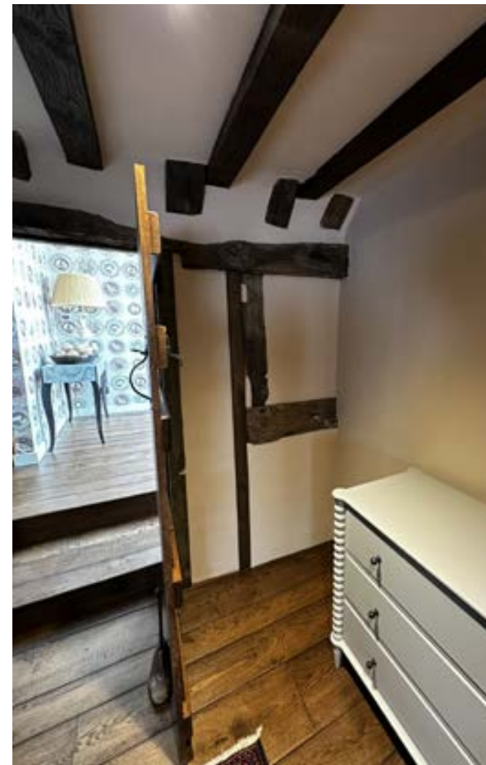
First Floor -step between existing house and extension (1997 planning approval)
