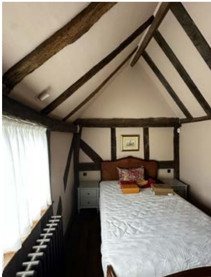
First Floor - historic timber frame roof
