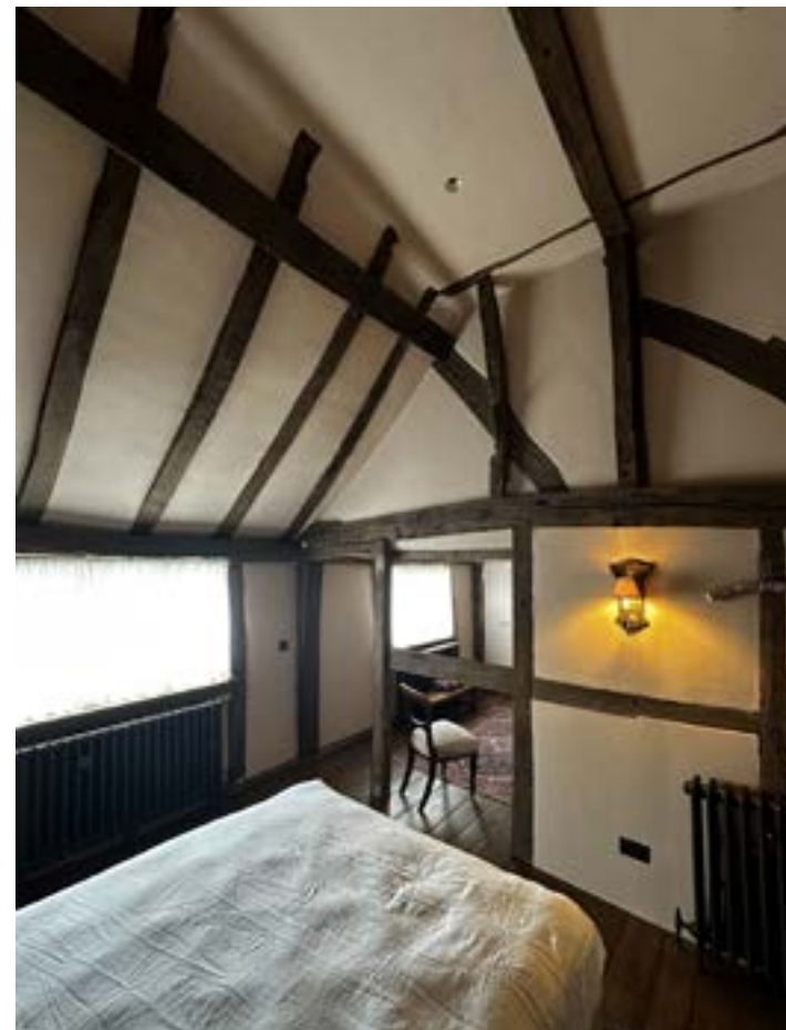
First Floor - historic timber frame roof
