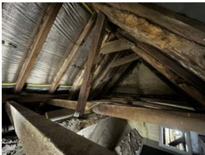
Attic - historic timber frame roof
