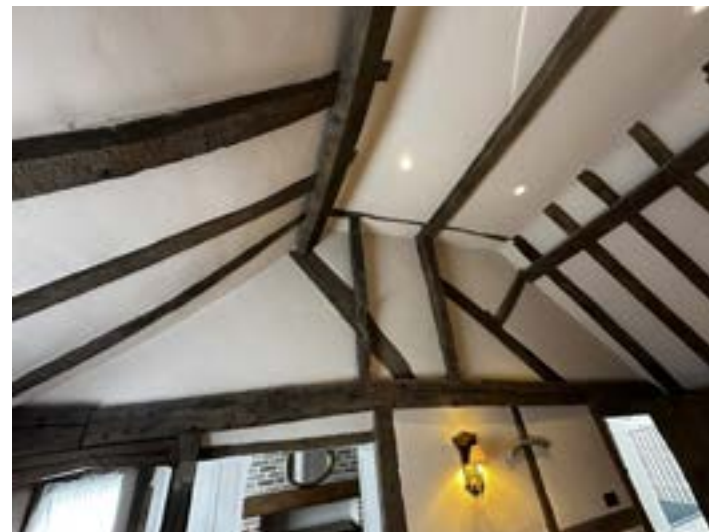
First Floor - historic timber frame roof
