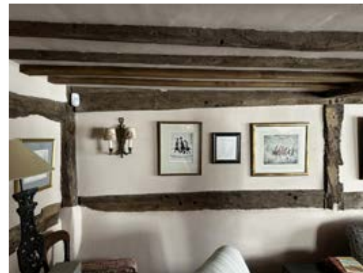
Historic timber frame wall, living room
