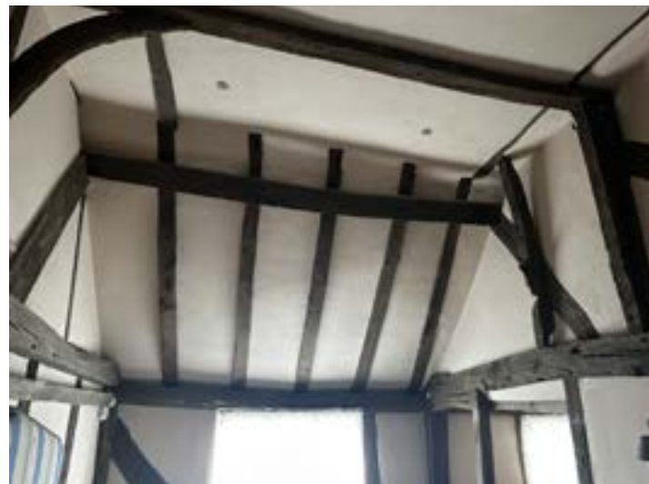
First Floor - historic timber frame roof
