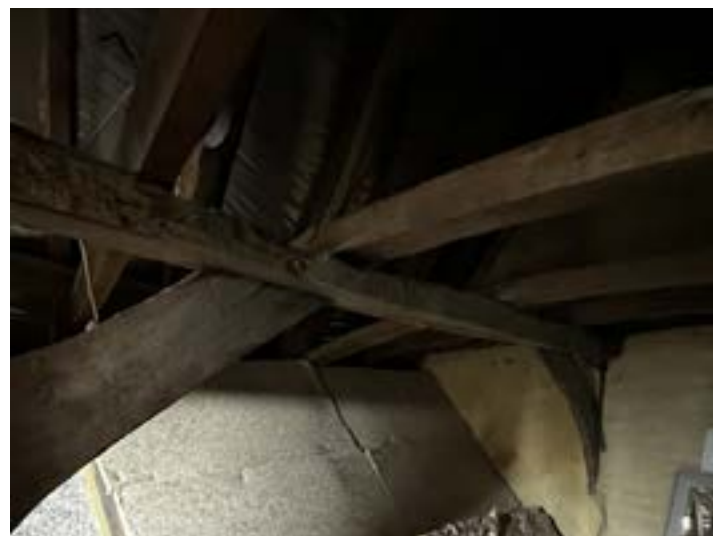
Attic - historic timber frame roof
