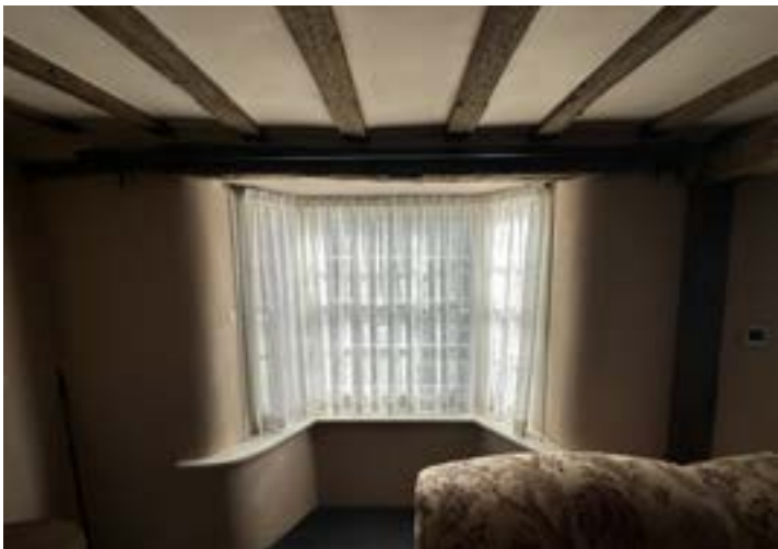
Ground Floor - living room bay window of re-fronted 19th century element of the building
