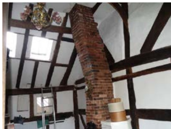
First floor bedroom, chimney stack
