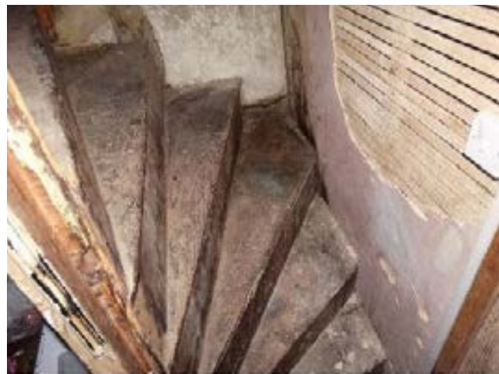
Corkscrew staircase - first floor (photograph taken during strip out pro)
