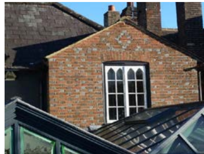
Historic rear extension with gothic window
