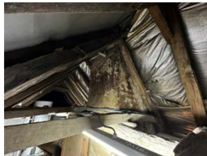
Attic - historic timber frame roof
