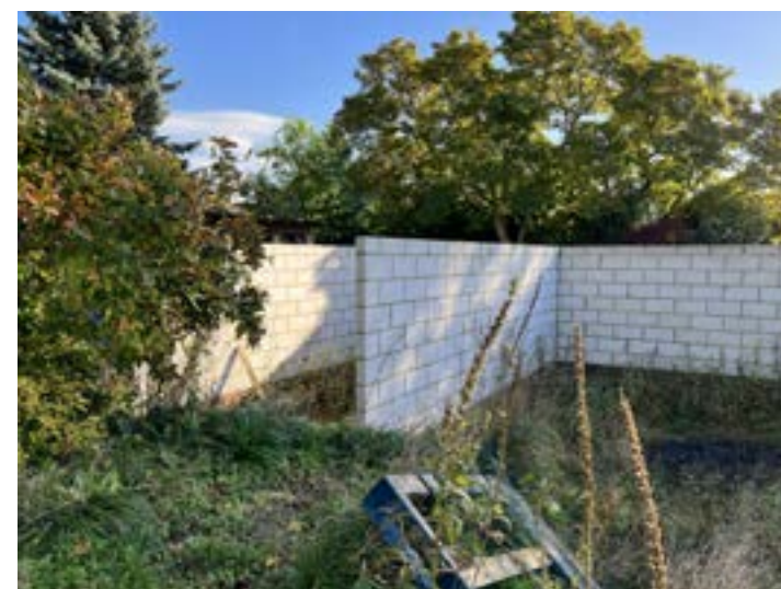
Garage walls constructed
