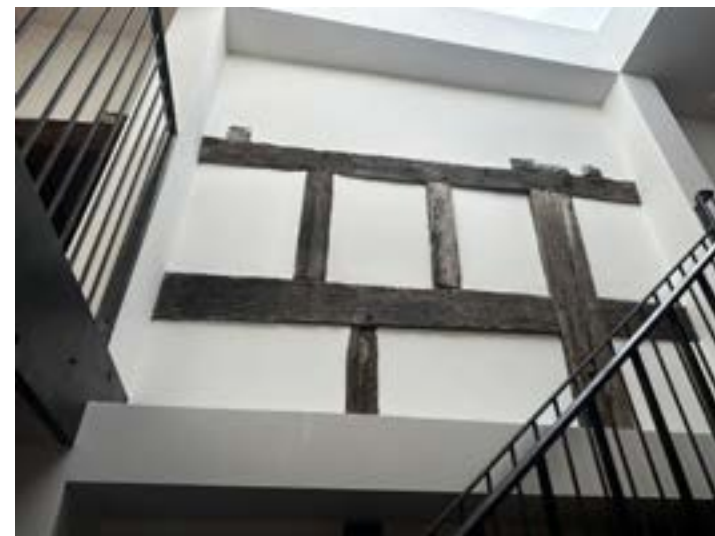
Historic timber frame wall in stairwell
