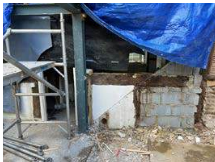
Breeze block within external and internal walls
