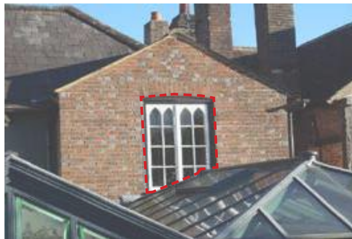
Pre-construction photograph - Victorian window, view from bedroom
