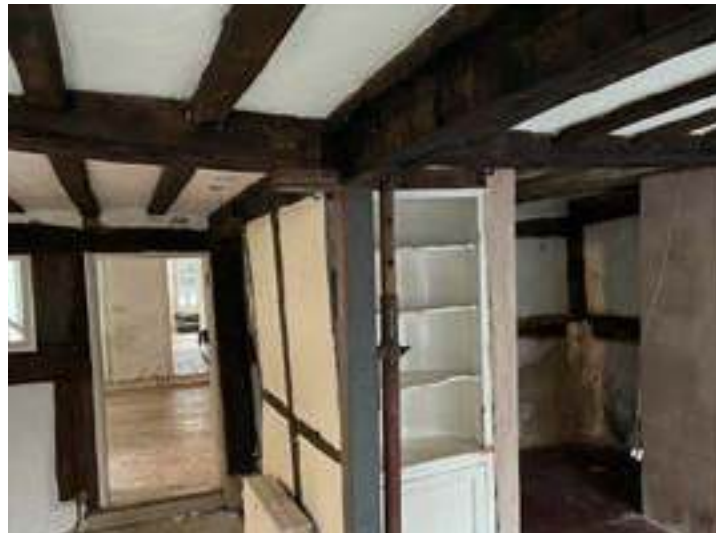
Internal wall and steel beam before removal
