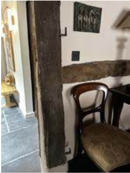
Photographs July 2025: historic evidence of a partition being installed in this location along with a door - the door hooks are still in place.
