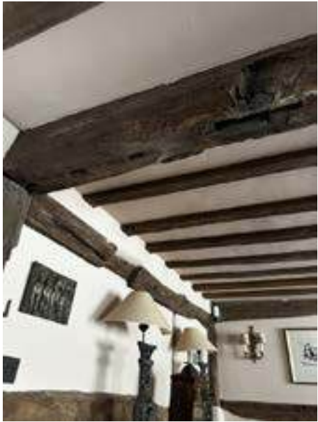
Photographs July 2025: historic evidence of a partition being installed in this location along with a door - the door hooks are still in place.
