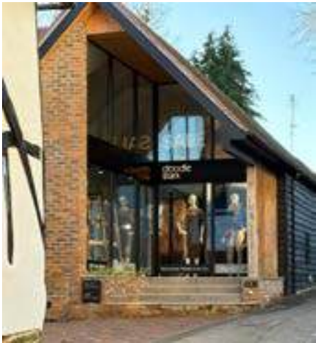
Local precedent: Doodie Stark shop, 66 High Street Lindfield (Listed Building) also historically a bake house
