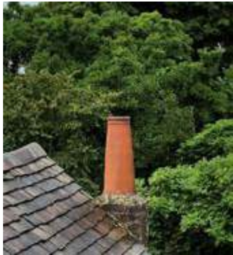
Original bake house chimney
