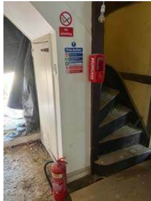
Staircase during demolition works
