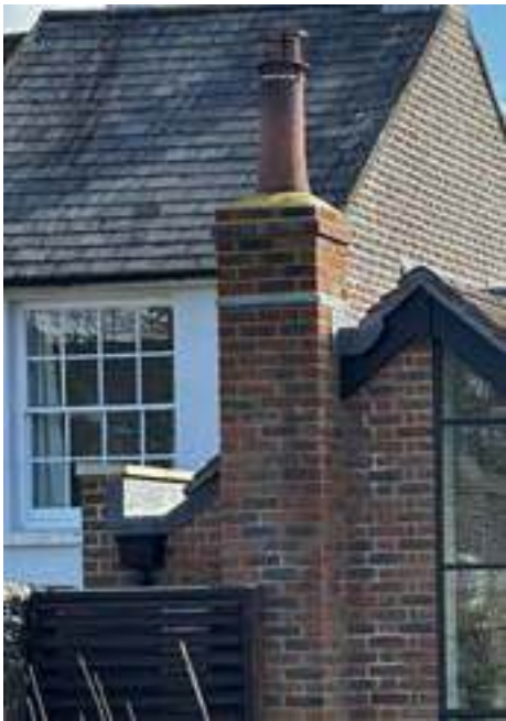
Recent photograph of parapet wall detail
