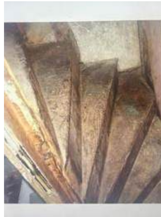
Staircase during demolition works
