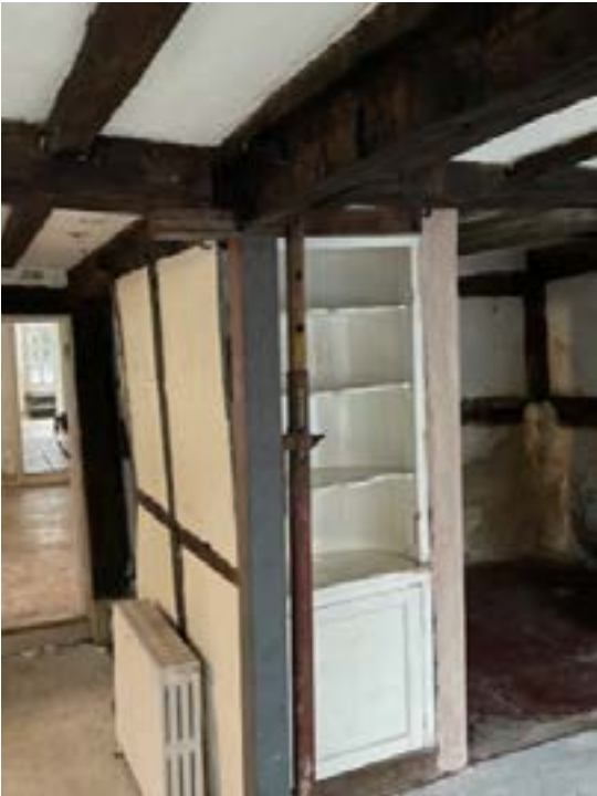
Pre-construction photograph - steel post supporting timber frame
