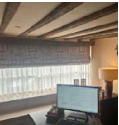
Photographs of ground floor study - previously not visible timber frame on ceiling exposed
