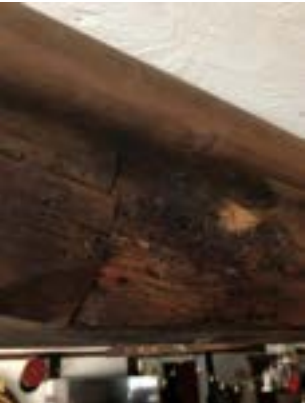
Photographs of oiled oak joist prior to restoration
