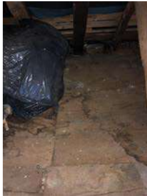
Pre-construction photographs of attic floorboards in poor condition
