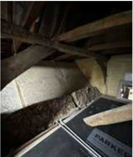
Attic, view of the vaulted ceiling Note retention of the original 17th century timber braces.
