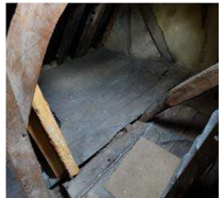
Extract from Desbrulais Heritage Report - area of attic floor with historic floorboards loose laid
