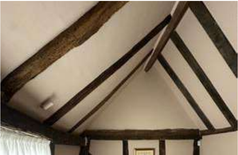
Vaulted Ceiling in SE Bedroom
