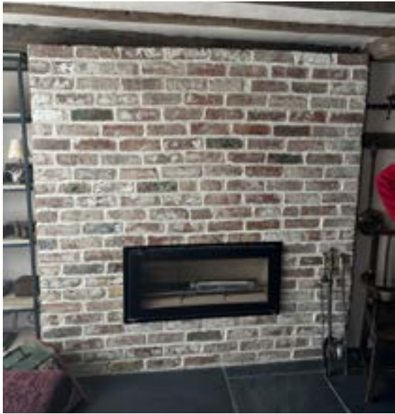
Ground floor living room re-faced chimney breast
