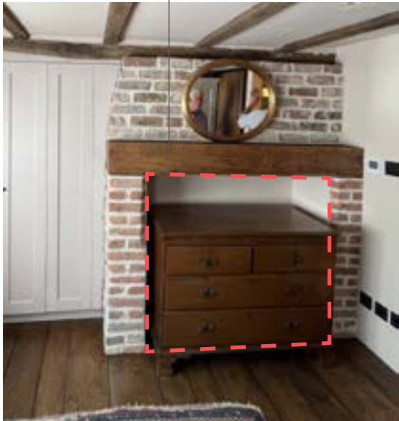
First floor bedroom re-faced chimney breast
