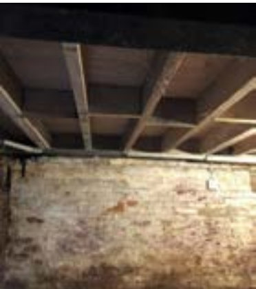
Pre-construction basement, railway steel member used for structural support, now replaced as per Structural Engineer proposal
