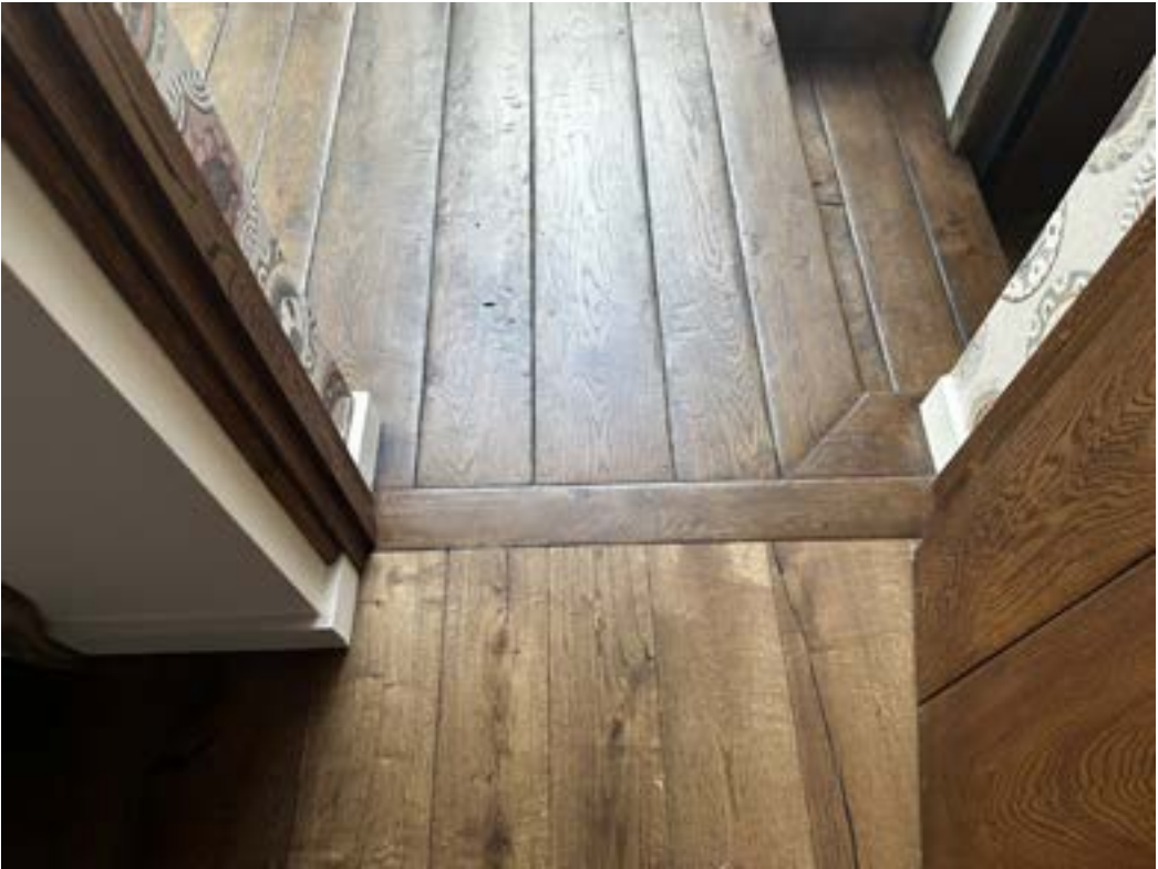
As-built oak flooring
