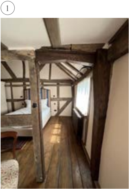
Photo of the doorway to the dressing room as implemented.
