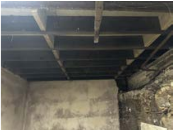
Basement, new softwood joists replacing rotten ones, brick wall finished with lime plaster, floor not altered.
