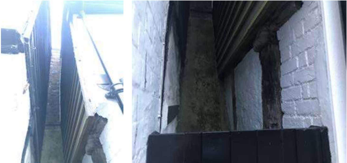
Recent photographs of timber weatherboarding
