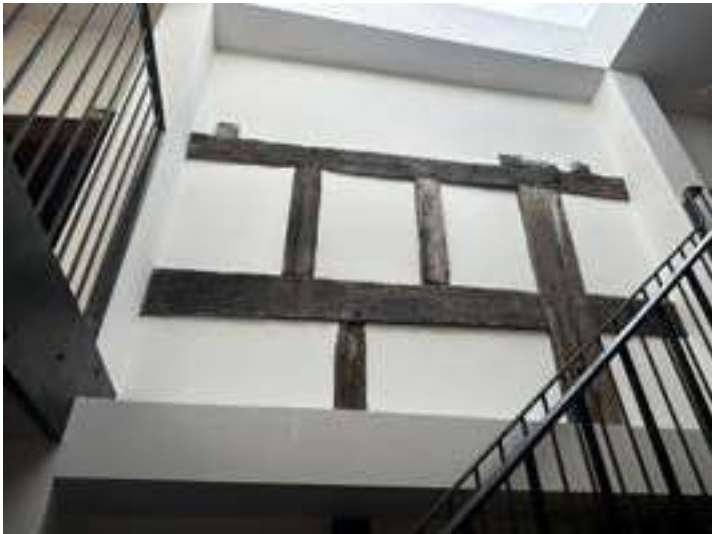
Recent photograph of west elevation wall with casement windows removed and openings filled in (first floor)
