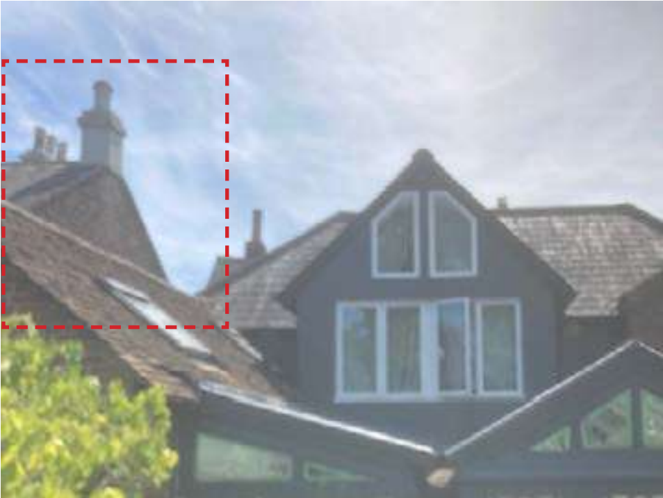
109 High Street south gable wall before re-pointing
