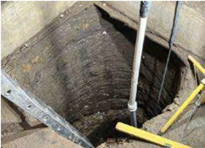
Opened well shaft
