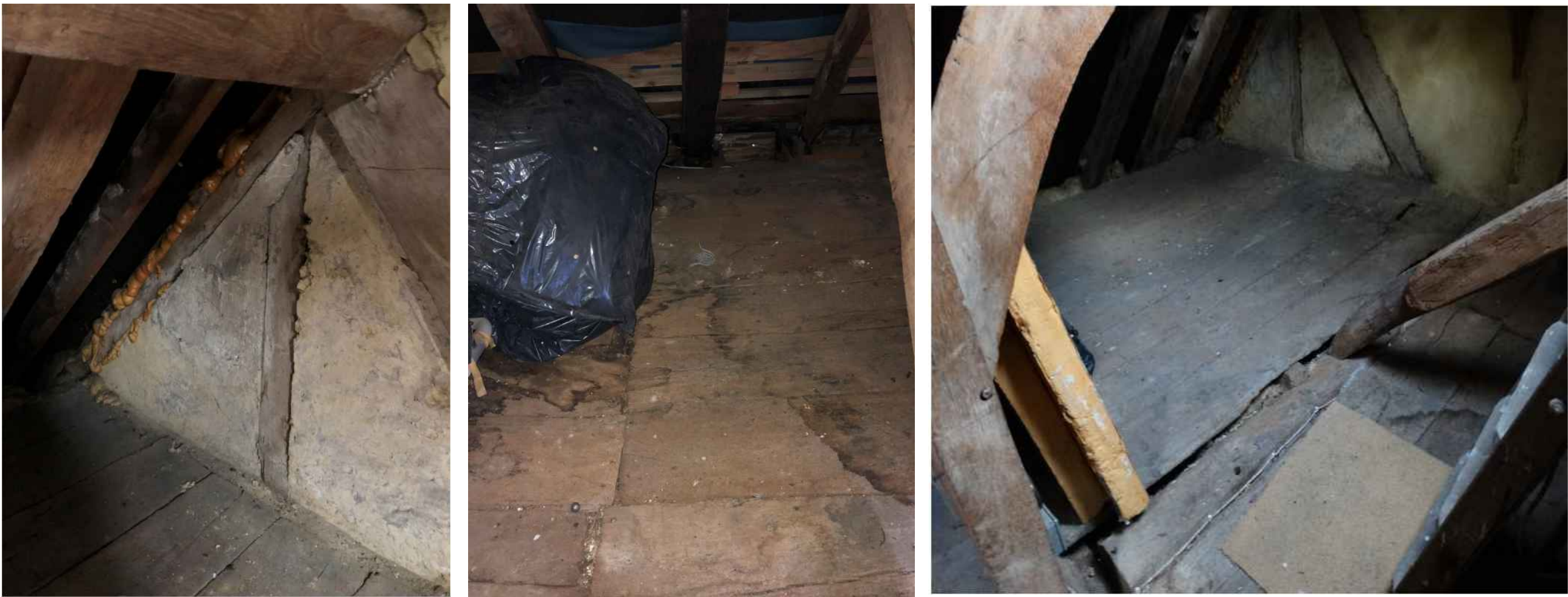
Pre-construction photographs of the existing attic floor boards in poor condition
