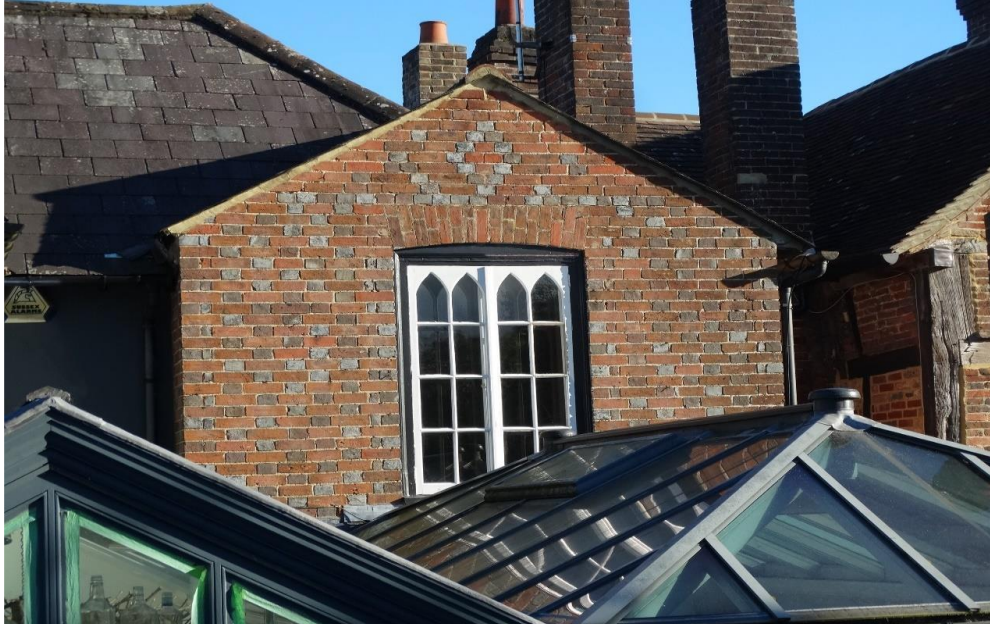
Figure 17: 1830s gabled outrigger with vitrified blue brick header detailing. N.B. the double casement window is mid C20 with inserted softwood spandrels suggesting a gothic pointed arch head. The original windows was likely an eight-over-eight vertical sliding hardwood sash. Source: Desbruslais Chartered Surveyors Statement of Heritage Significance of 13 th October 2022
