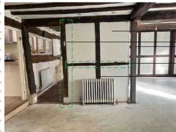
Internal lounge wall prior to changes.
