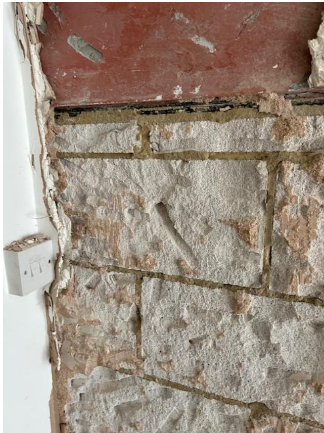
Figure 37: Blockwork construction underlying the cosmetic 'timber stud' wall with stonework nogging shown at Figure 16
