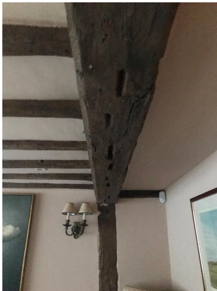
Figure 13: N-S ceiling beam to the former dining room to the south bay with mortices indicative of historic partitioning within this space.
