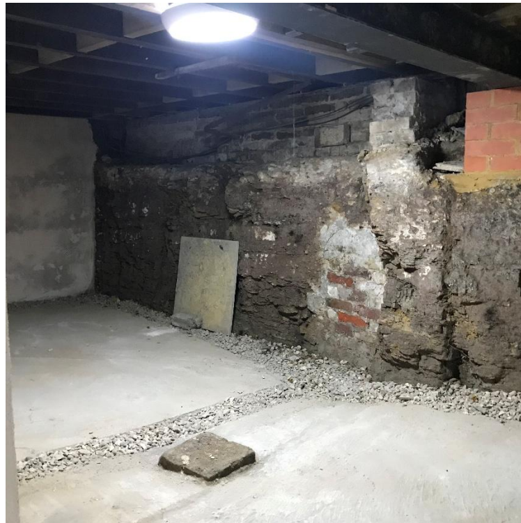
Figure 36: Renewed steel beam with new nogging and joists at basement level. The pre-existing concrete floor has been augmented by a French drain and brick walls coated with breathable hydraulic lime render to regulate the damp.
