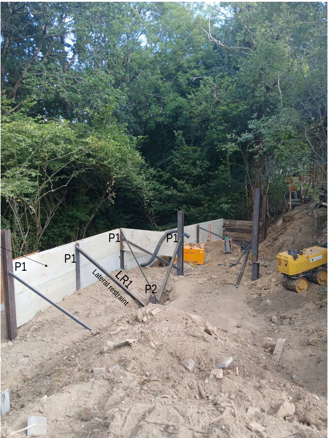
As-build during construction showing RW1 comprising 2 no 3m x 1m concrete planks set into webs of P1 and braced/laterally restrained onto top of P2
