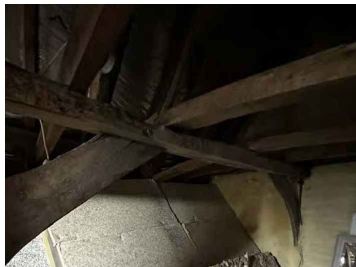
Attic - historic timber frame roof
