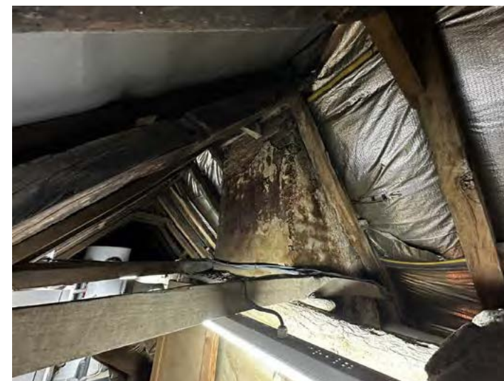
Attic - historic timber frame roof
