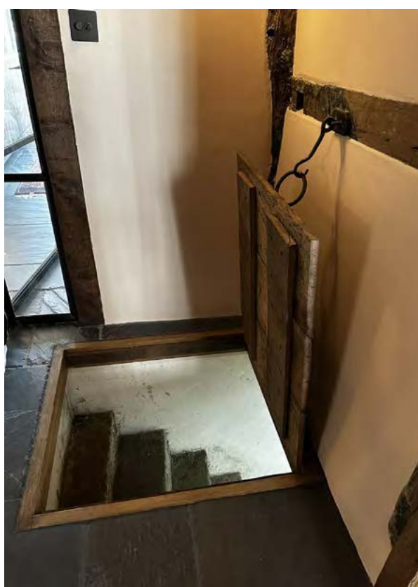
Ground Floor - access hatch to basement
