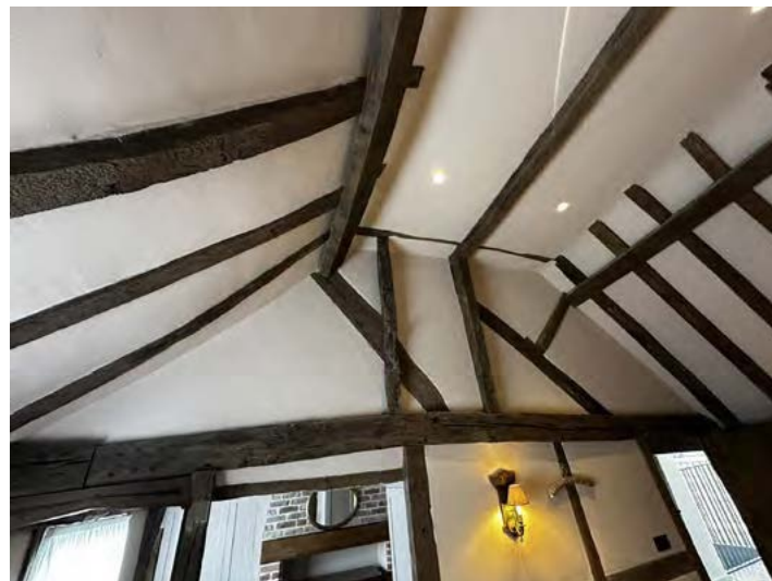
First Floor - historic timber frame roof
