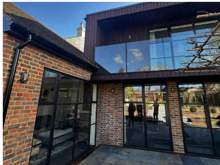
Rear elevation & re-constructed bake house
