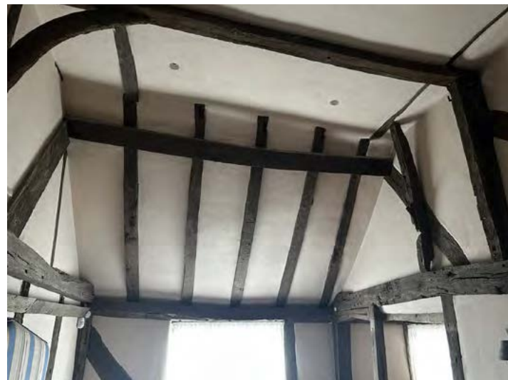
First Floor - historic timber frame roof
