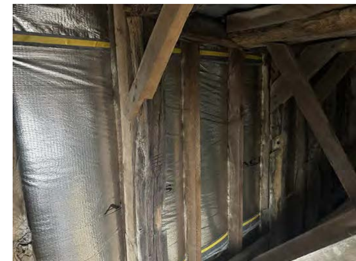
Attic - historic timber frame roof, new insulation
