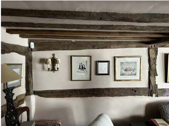
Historic timber frame wall, living room
