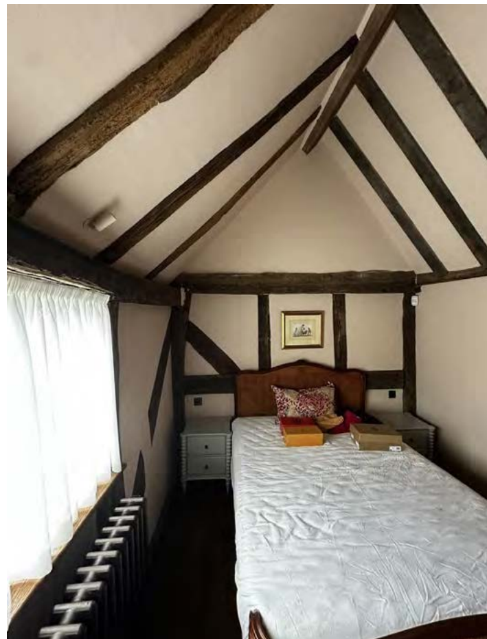
First Floor - historic timber frame roof
