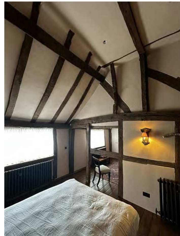
First Floor - historic timber frame roof
