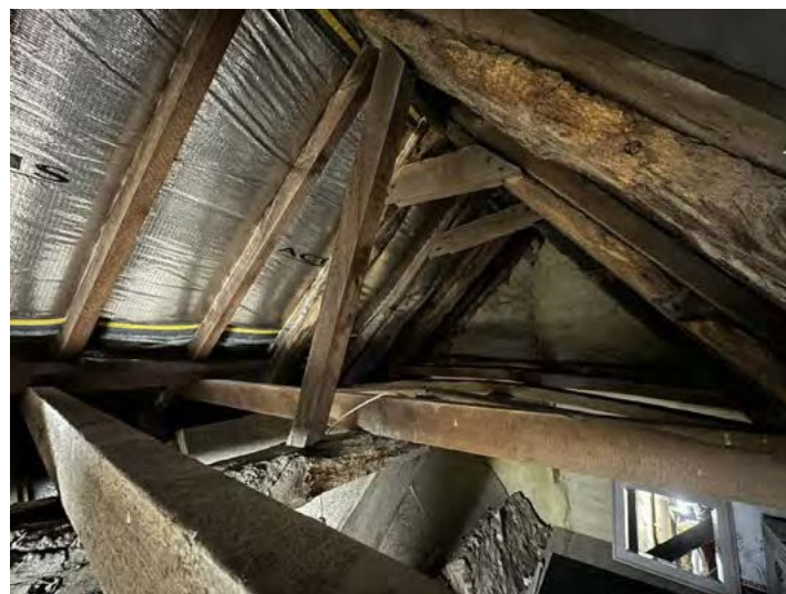
Attic - historic timber frame roof
