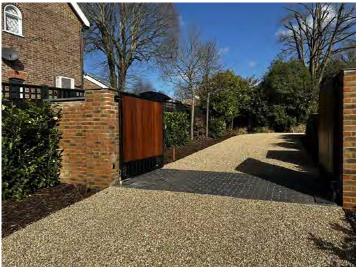
Gravel driveway and new gates
