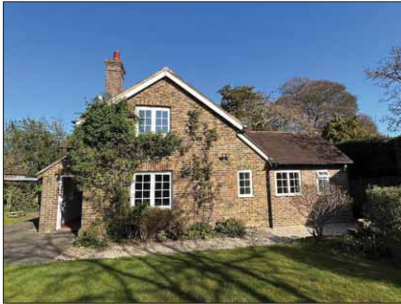
Image 11: Highbrook Cottage, southeast facing elevation
