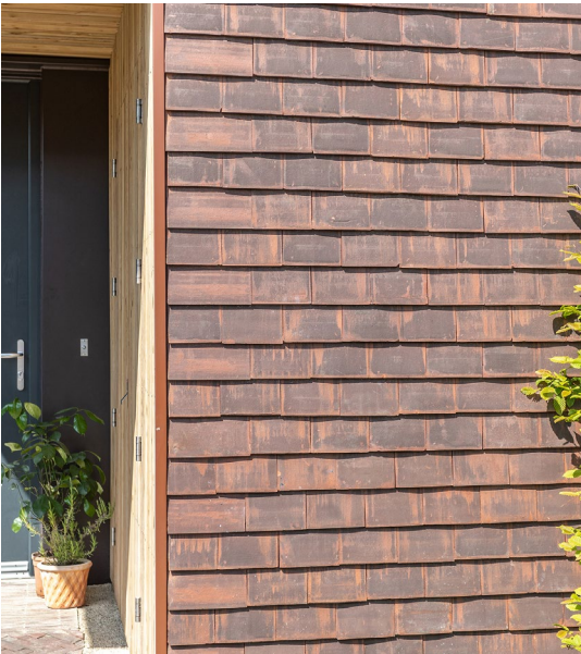
2. WALLS (UPPER) - CLAY TILE HANGING
