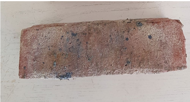
1. WALLS (LOWER) - LOCAL STOCK BRICK
