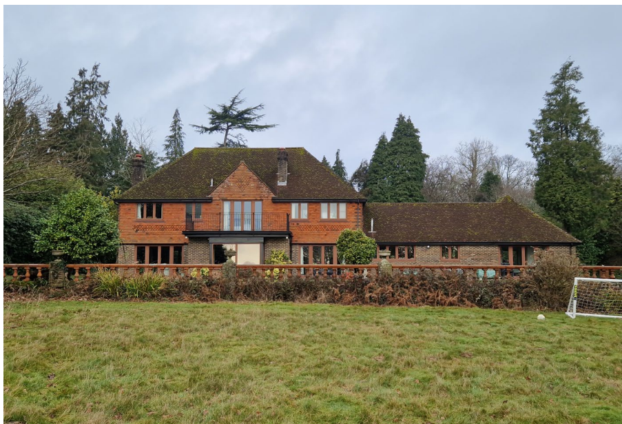
2. View of rear elevation
