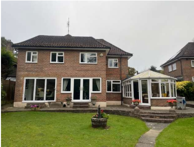
View looking west showing rear elevation
