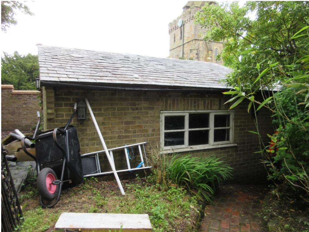
Figure 6: West elevation of the garage in the rear garden of the Site.
