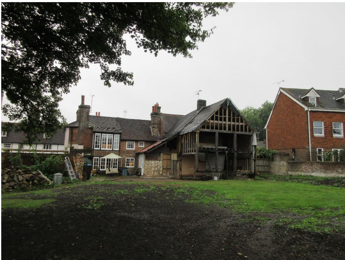
Figure 3: Rear elevation of The Friary, Somners and Dumbrells, and the rear garden (westward view).
