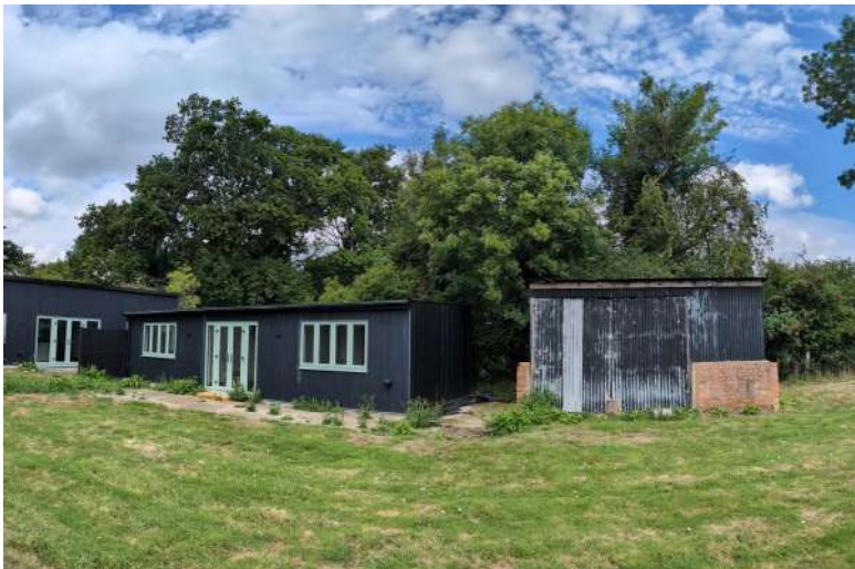
Photo 2: Trees to rear of existing structures.
