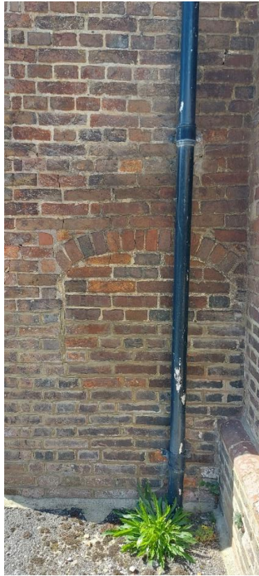
Plate 3. Former window/coal chute doorway on southern side of the building.
