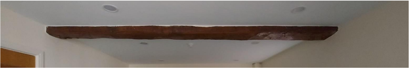
Plate 7. Ground floor roof beam at western end.
