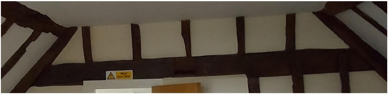
Plate 13. Upper floor cross beam.
