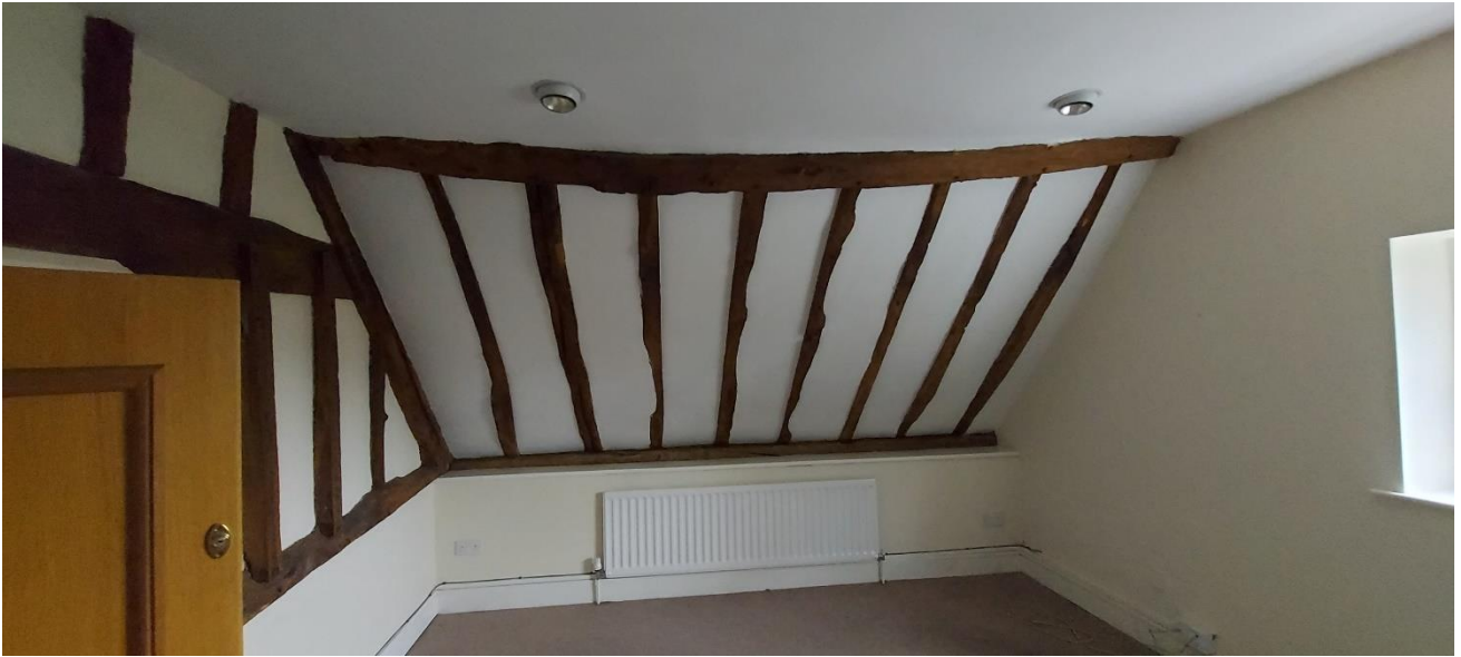
Plate 11. Mediaeval beams set into modern plaster.
