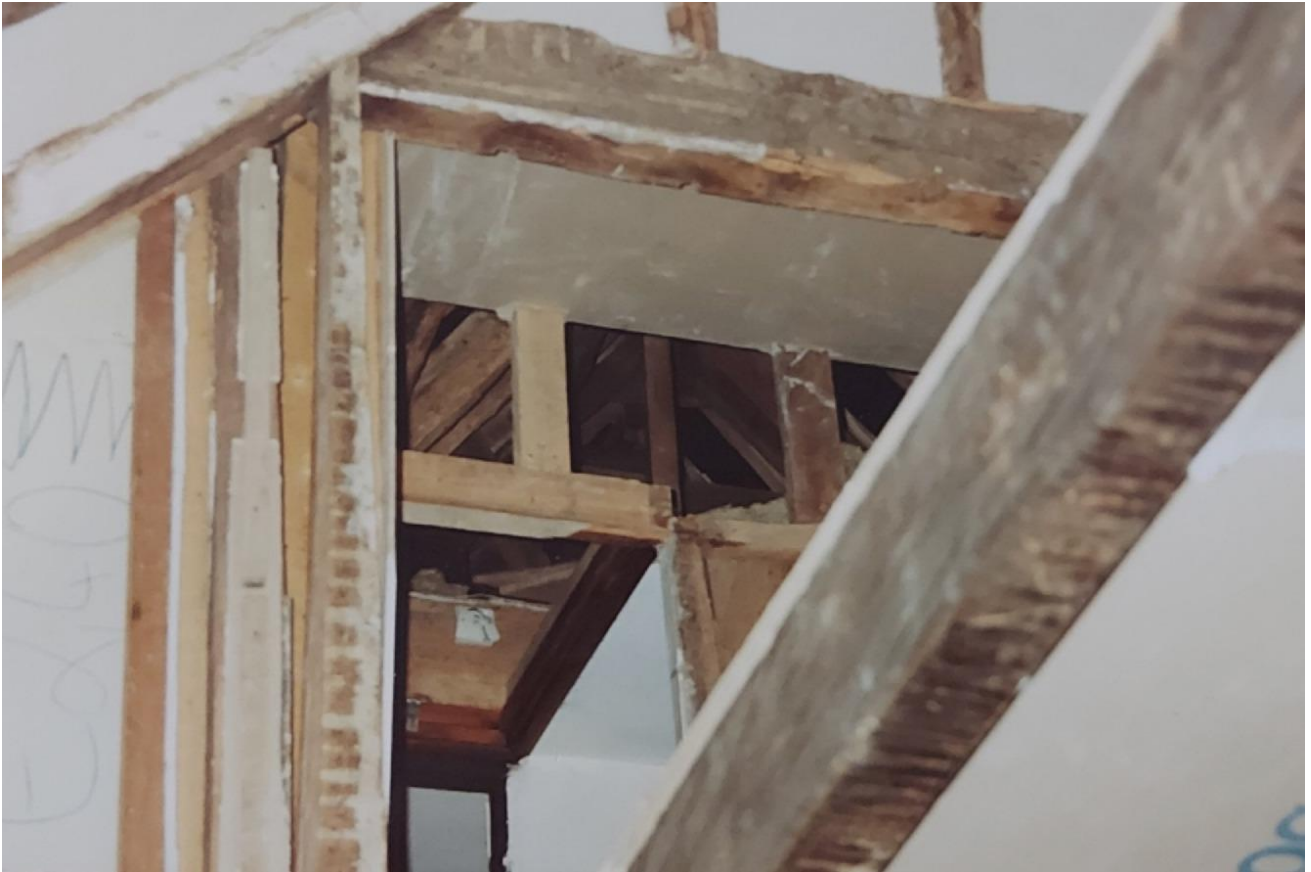
Plate 17. New timbers being installed during renovation work of the 180's or 1990's.
