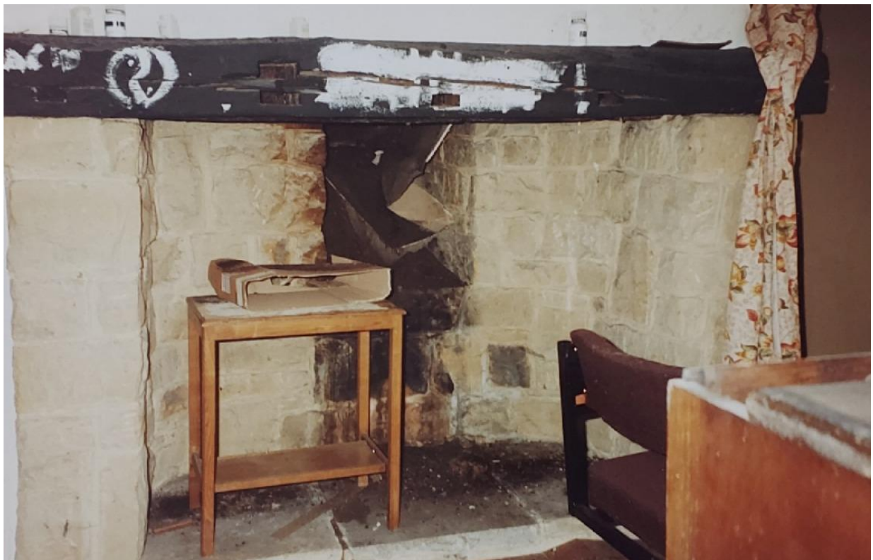
Plate 6. Ground floor fireplace during renovation works of the 1980's or 1990's.
