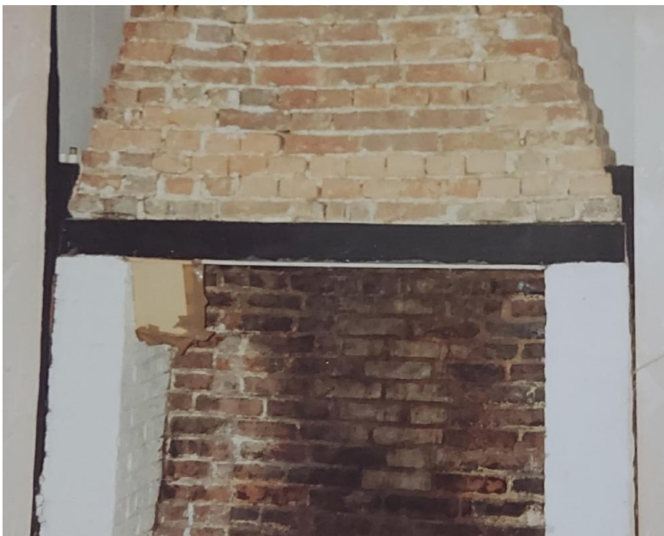
Plate 16. First floor fireplace during renovation works of the 1980's or 1990's.
