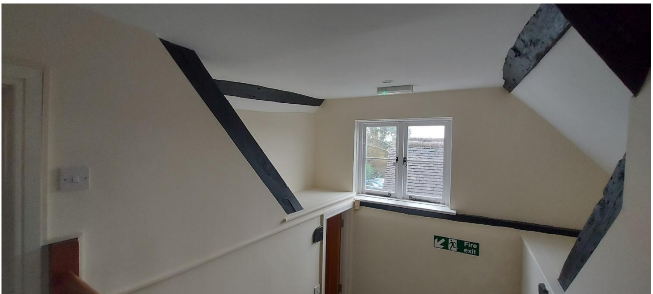
Plate 10. Stairwell construction beams.
