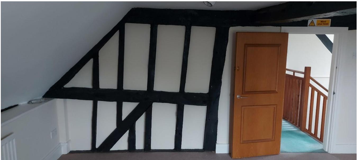
Plate 12. Upper floor box frame construction beams.
