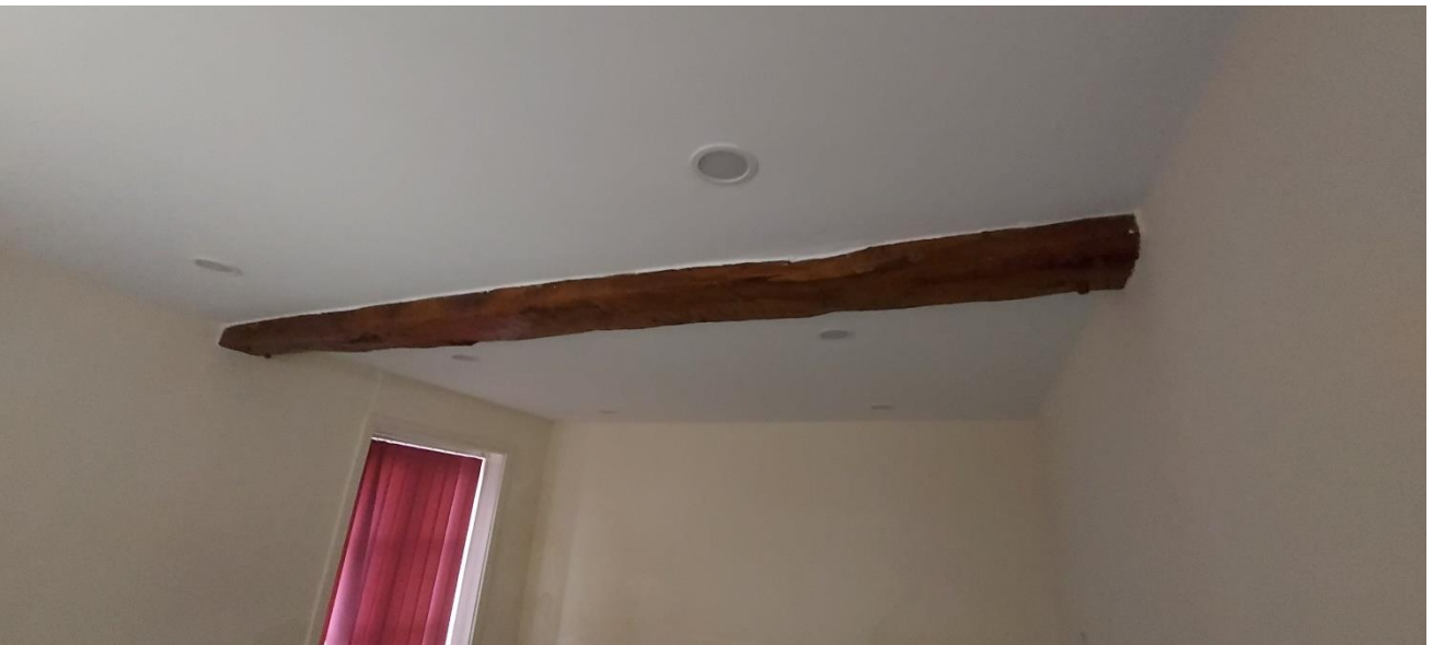
Plate 8. Ground floor roof beam at eastern end.
