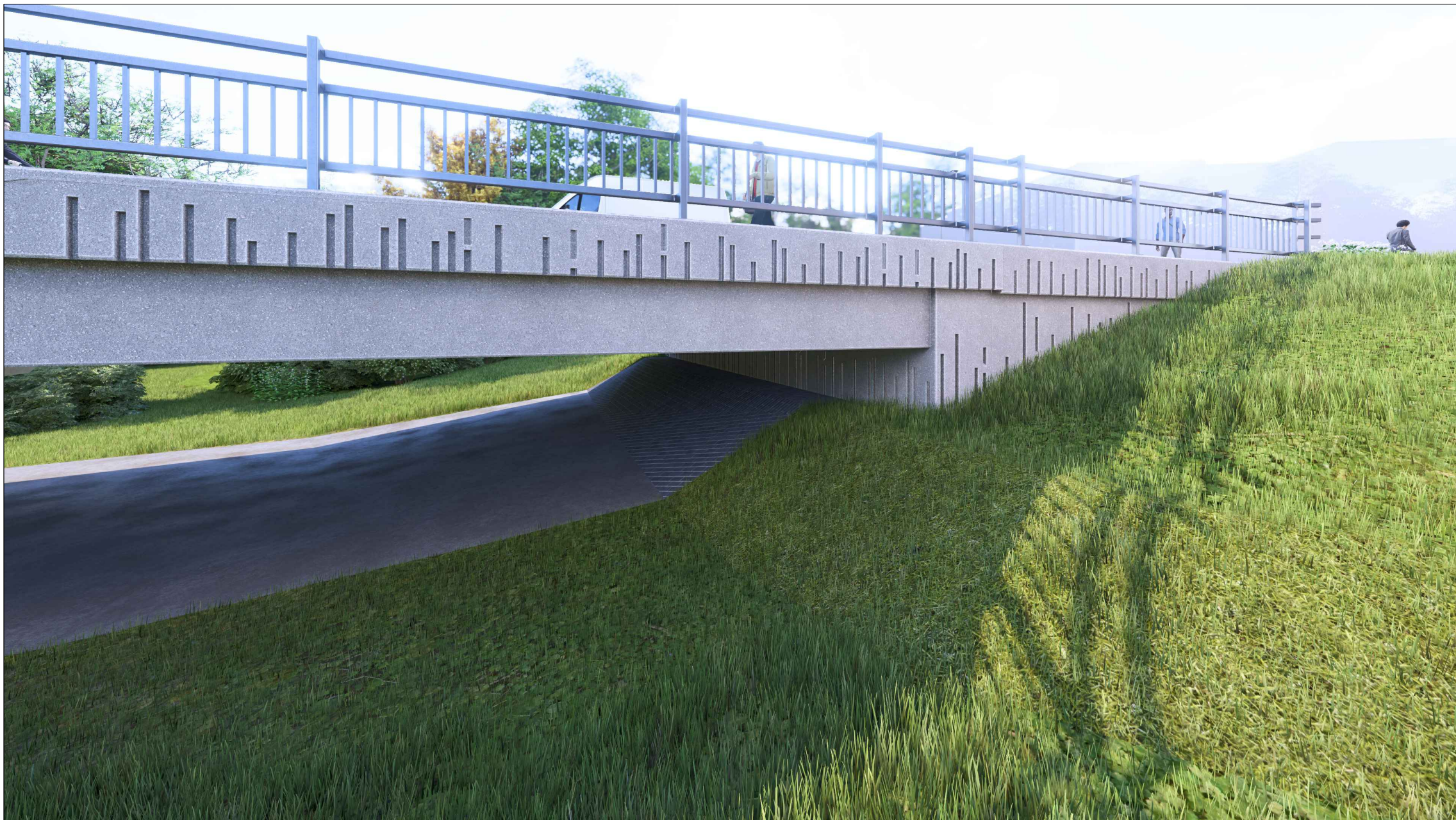
VIEW OF THE EAST ABUTMENT
