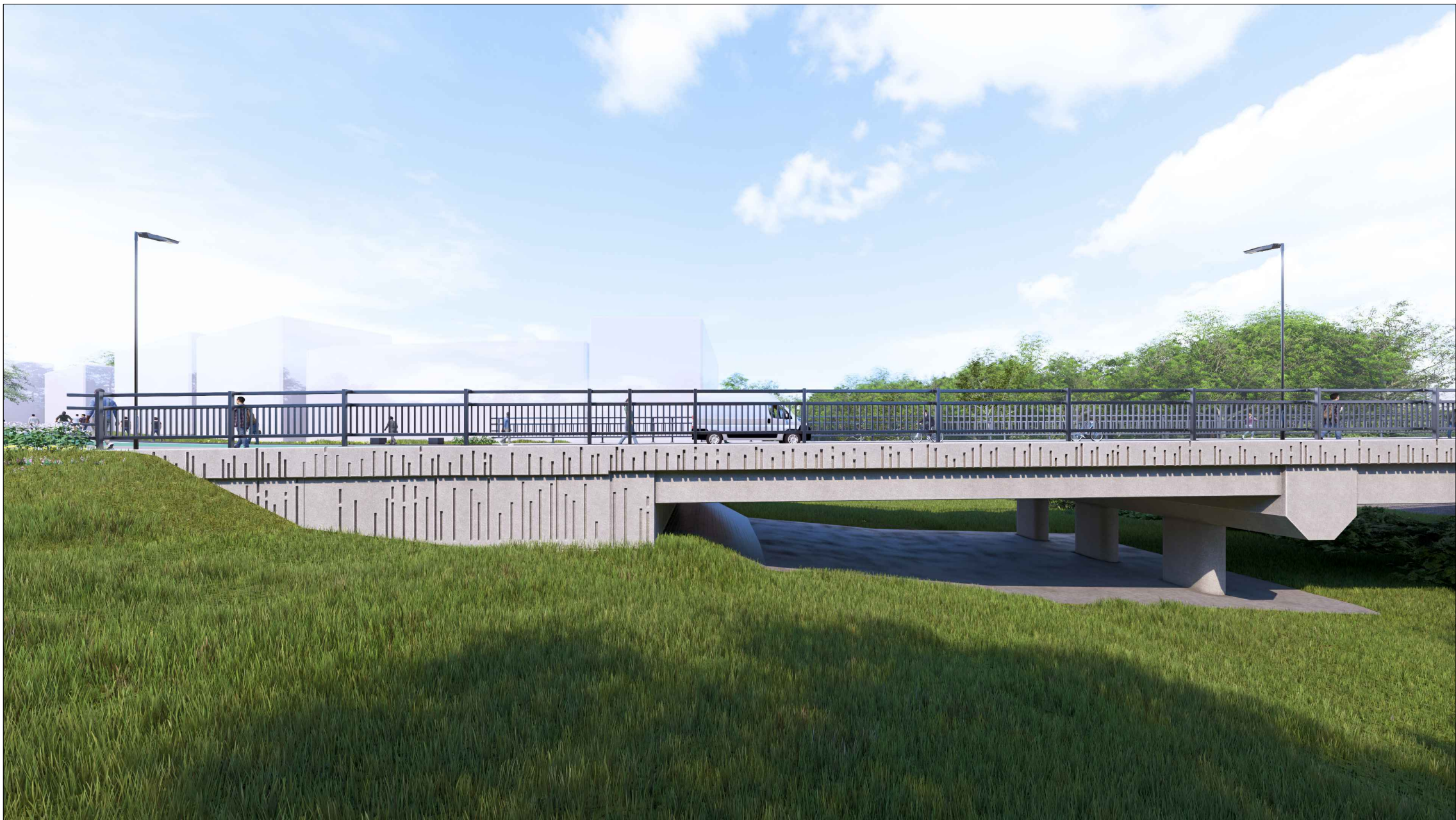
VIEW OF THE EAST ABUTMENT AND NORTH EAST RETAINING WALL
