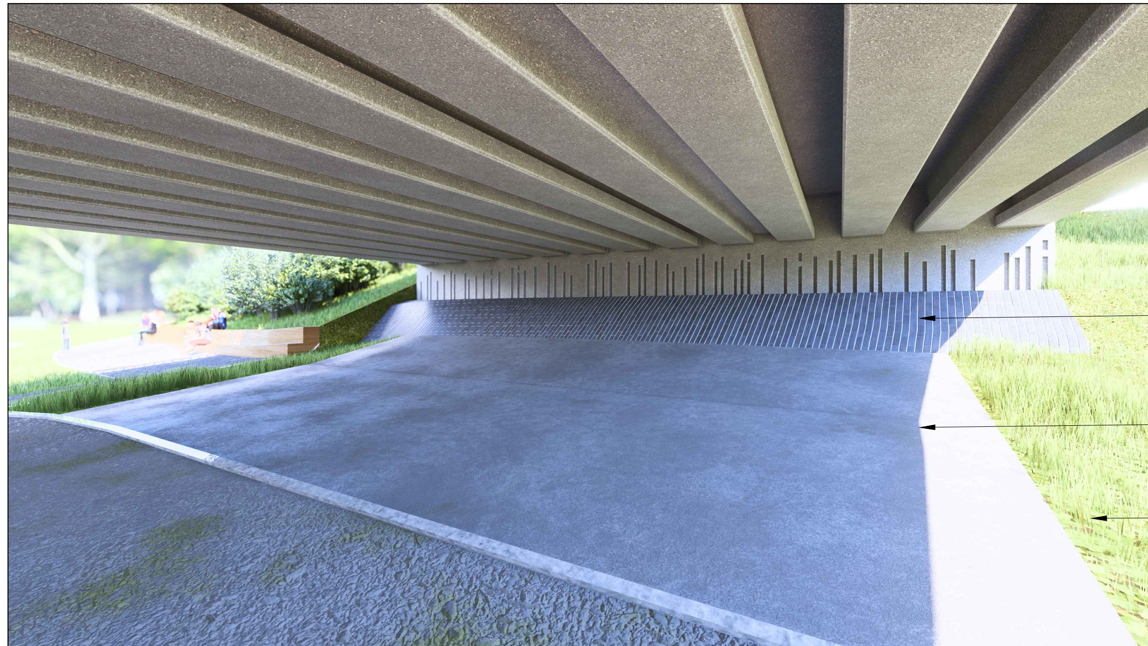
VIEW OF THE WESTERN ABUTMENT
