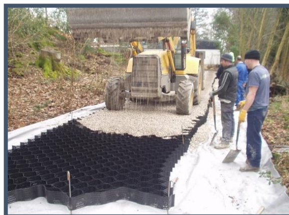
Figure 12 Examples of Cellweb filling with angular stone
