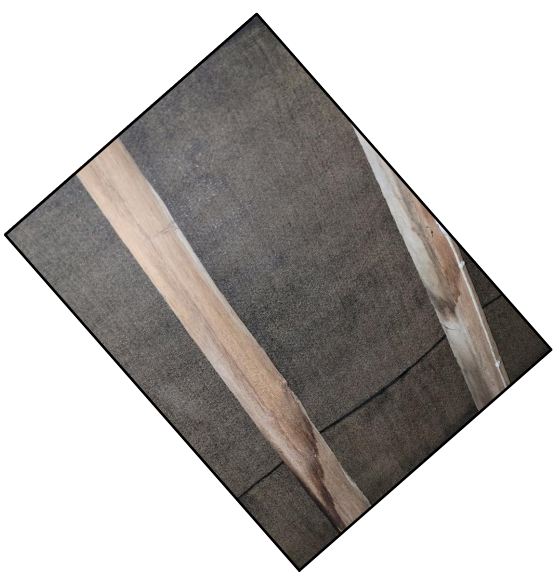
RAFTERS AT ROOFLIGHT 2
