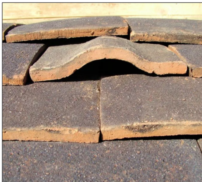
Figure 6. (Left) Example of bat access tile, available from www.nhbs.com
