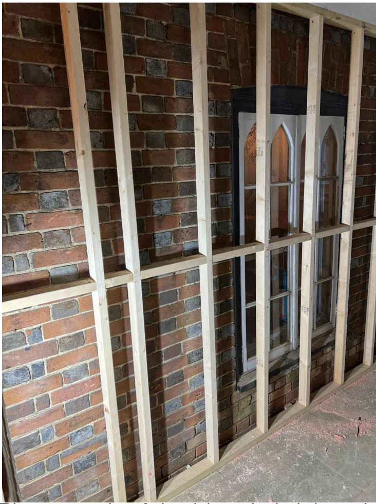
Photograph of the historic brickwork gable wall before it was covered
