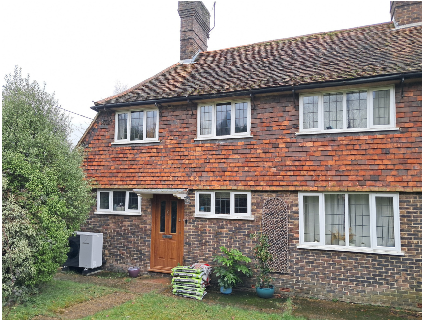
Front Elevation – general view
