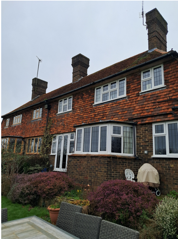
Rear Elevation – general view
