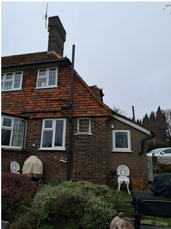
Rear Elevation – general view
