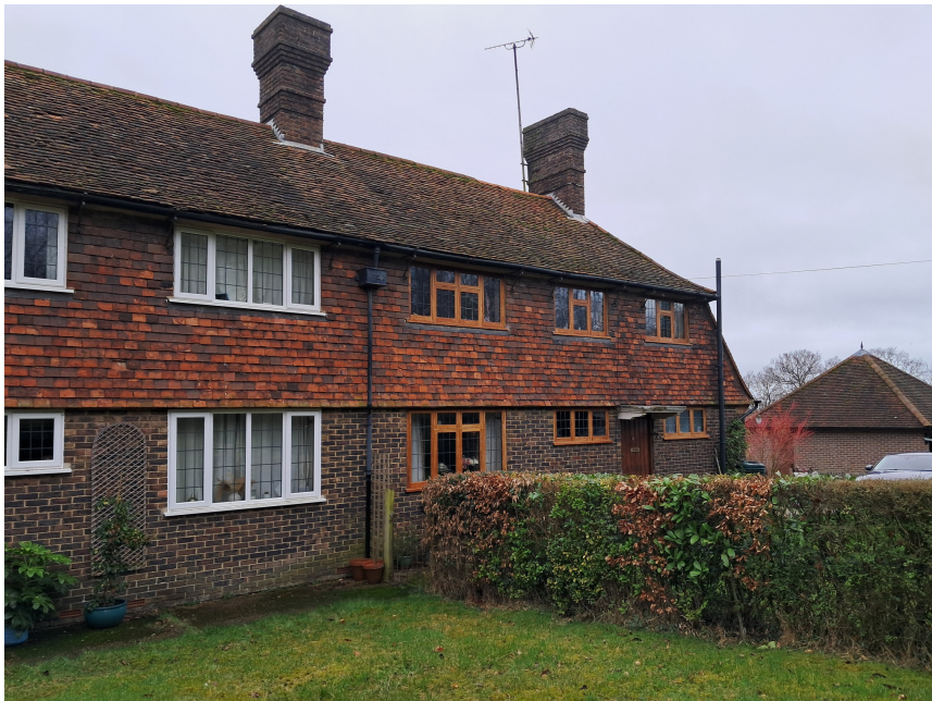
Rear Elevation – general view
