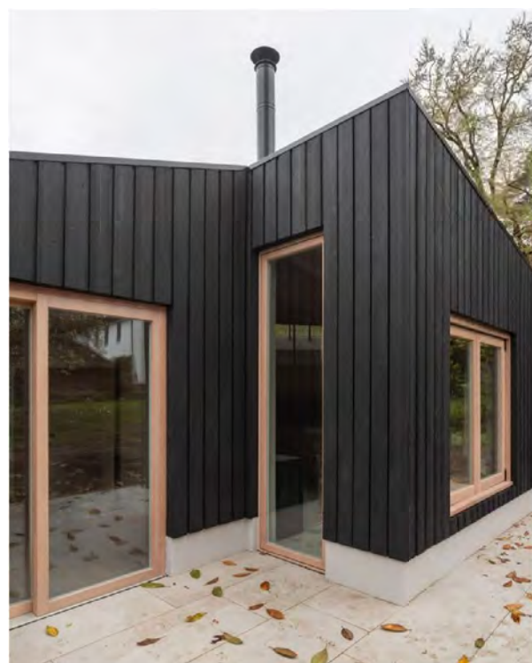
Metal cladding with stained timber accents
