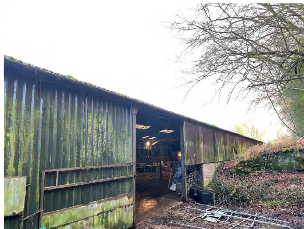
Current Barn - dark green cladding, natural timber and concrete blocks
