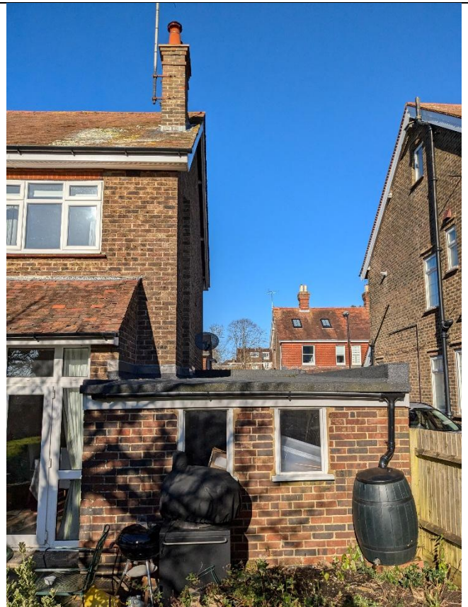
Existing rear elevation of existing flat roof garage extending into garden
