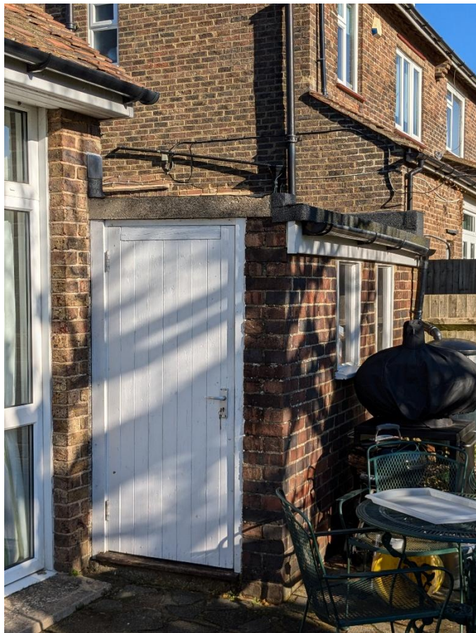
Existing rear elevation - Garage Access
