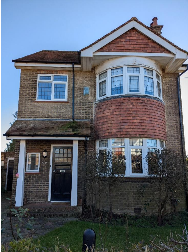
Front elevation of 52 Crescent Road
