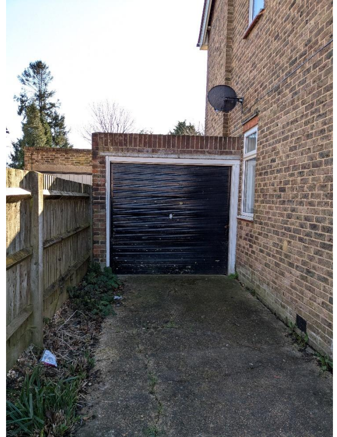
Existing front elevation of flat roof garage
