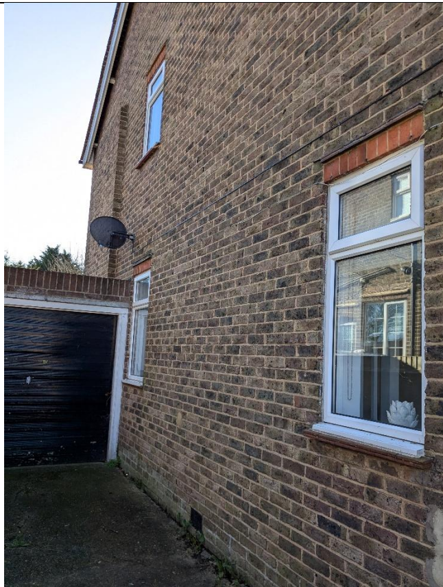
Existing side elevation showing garage
