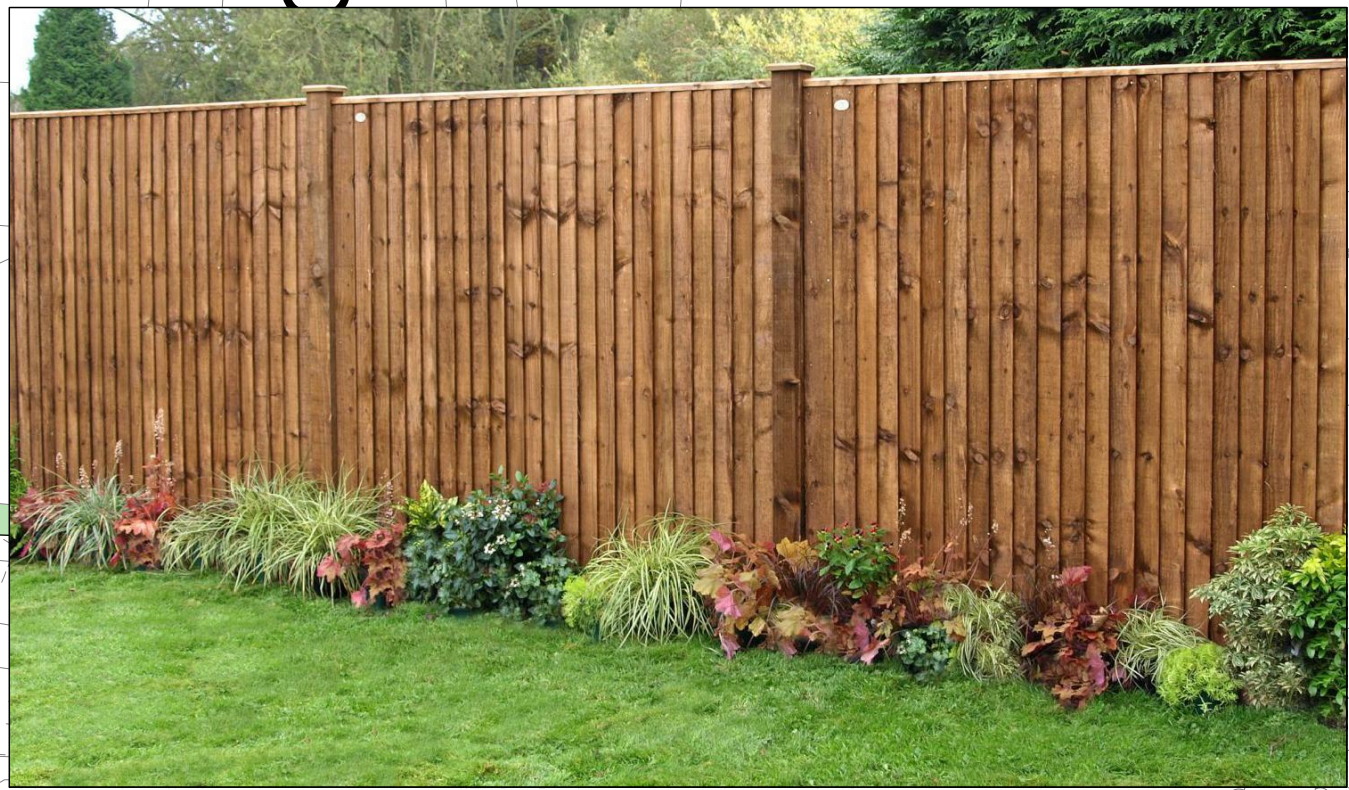
1.8m HIGH CLOSE BOARD FENCE. Typical fencing used for all plot and site boundary
