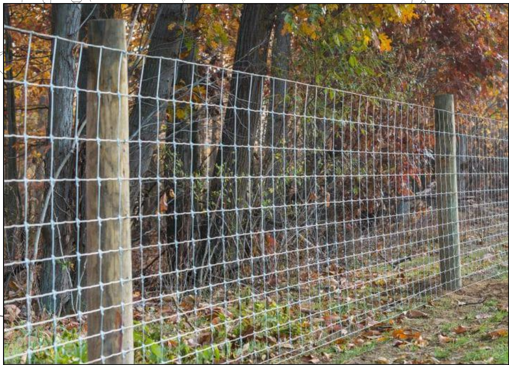
1.0m HIGH POST AND WIRE. Site boundary to rear of Ecology Zone
