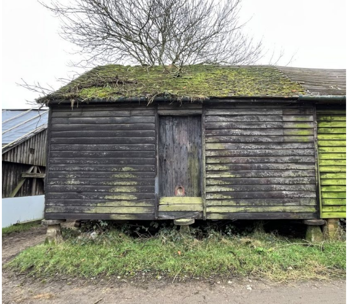
Figure 4: Building 5, North Elevation (January 2025). 19 th century staddle stones hold up the timber framed granary
