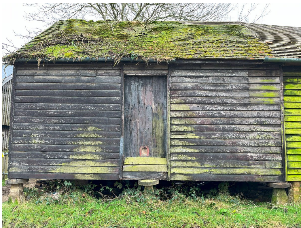
Figure. 11. North Elevation of Granary with raised entrance door but no steps up to it, abutting a much later extension on brick piers. (January 2025)
