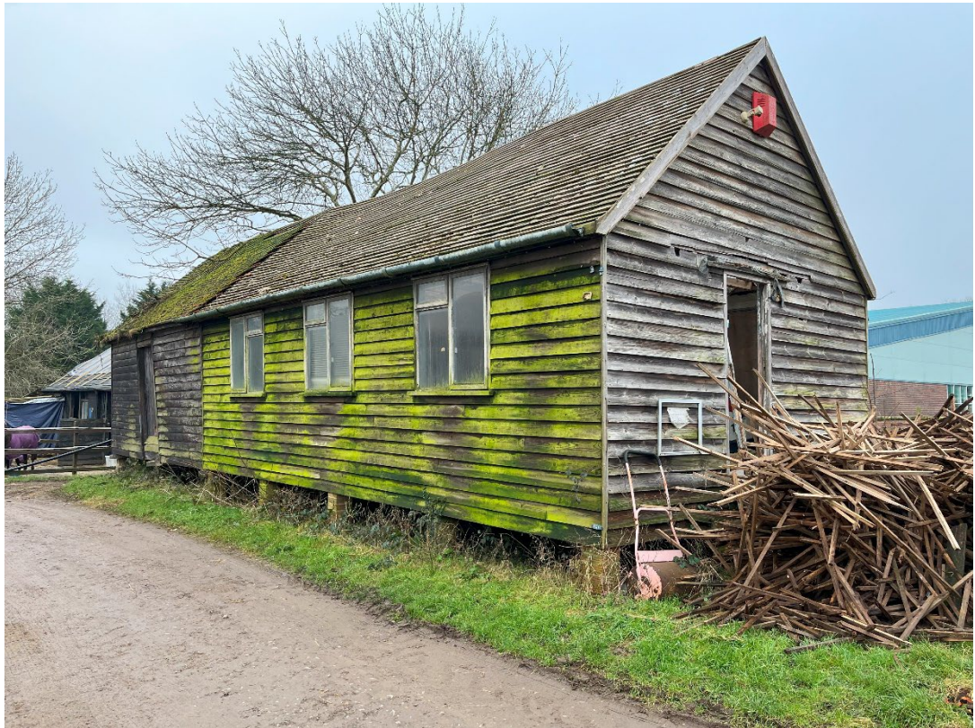
Figure 1: Building 5 or Site Office (January 2025)
