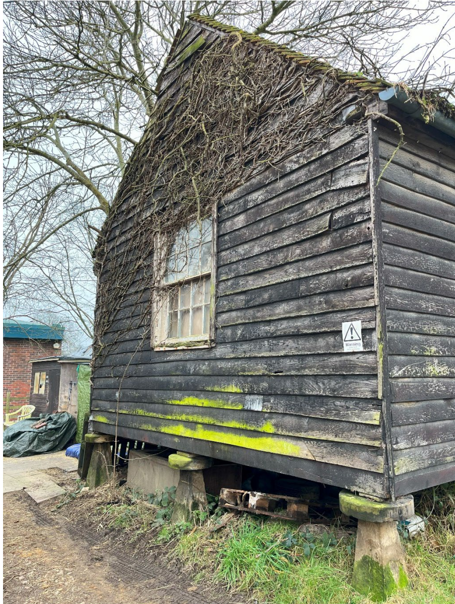
Figure. 12: East elevation of granary with likely later inserted Georgian window (six over six sash with no horns). (January 2025)
