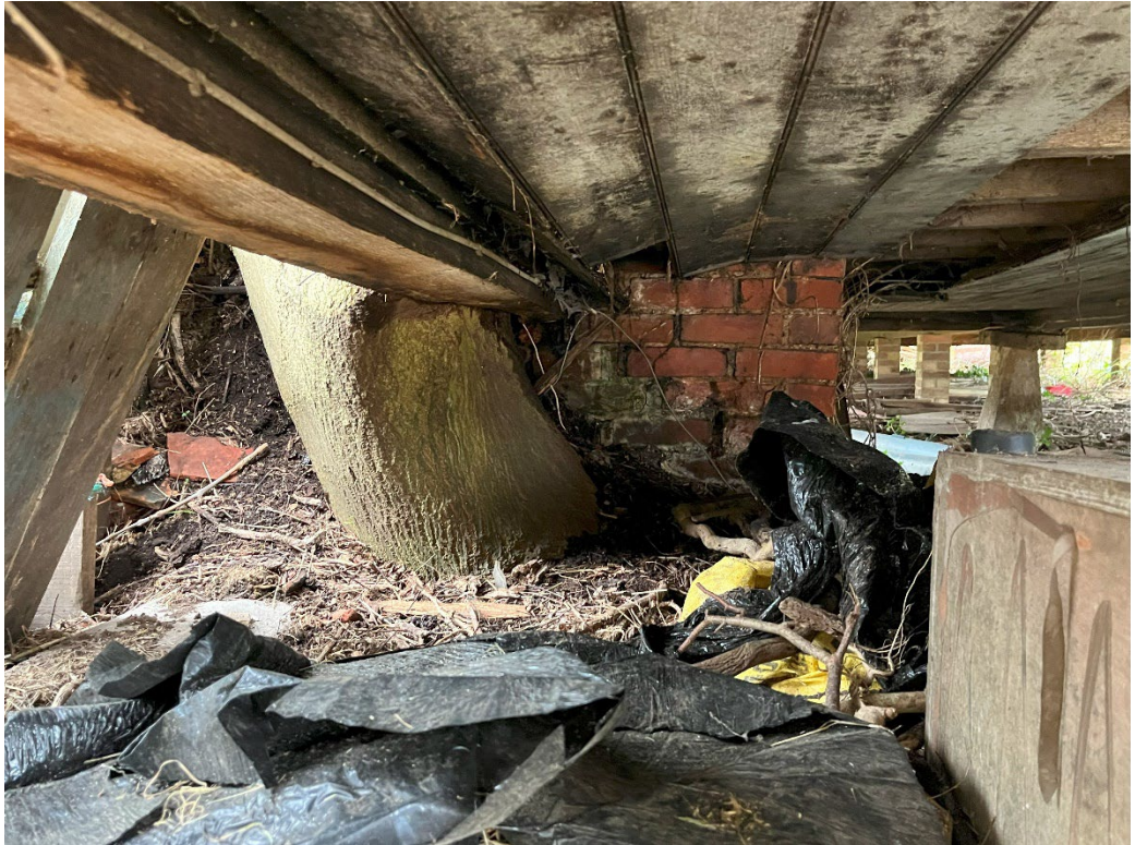
Figure 14: View of tree and chimney stack base under existing granary looking west (January 2025).
