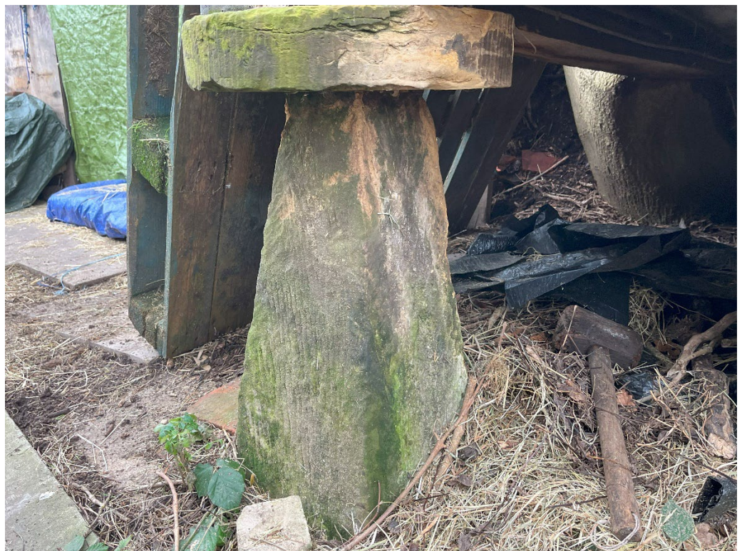
Figure 15: Existing staddle stone, southeast corner, one of 9. (January 2025)
