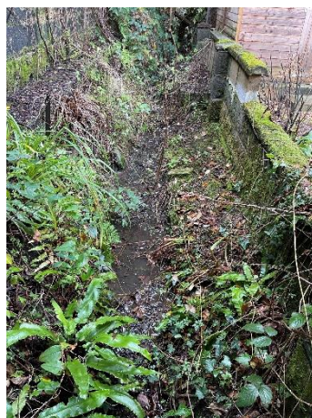
Fig 02 – the main body of the ditch
