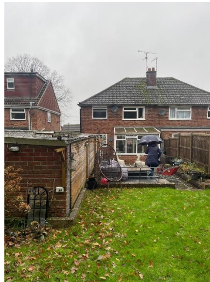
Rear Elevation (showing conservatory and garage to left – both to be demolished)
