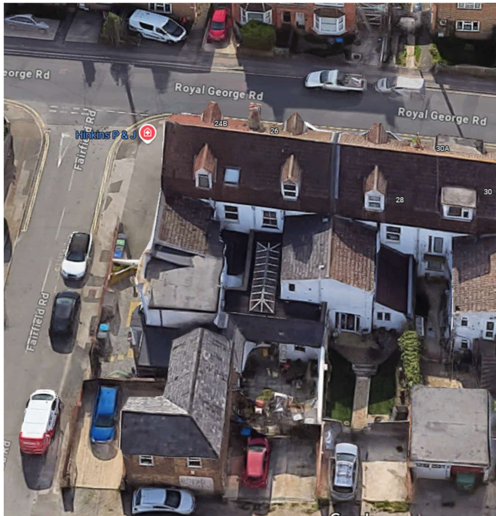
Figure 3: Aerial view of the building
