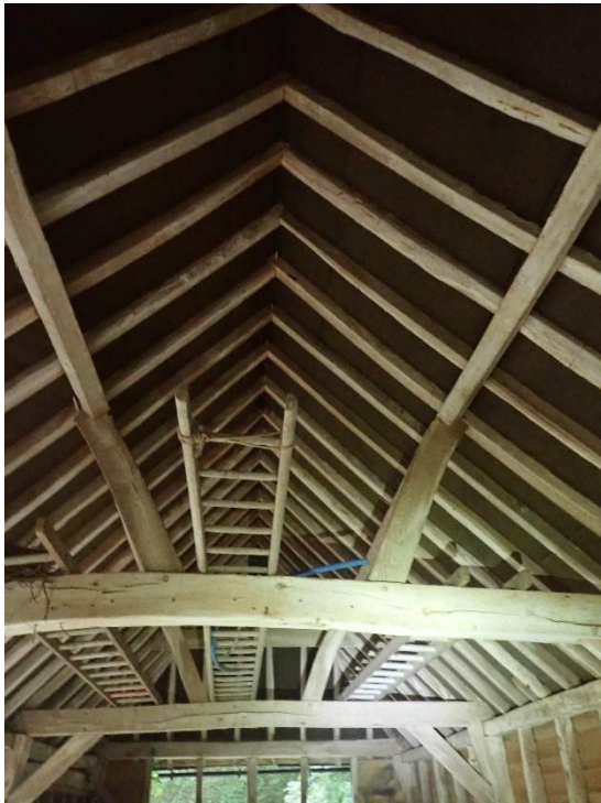
Fig. 8 – View S along interior of barn roof
