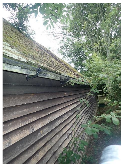
Fig. 4 - Rear (W) side of barn
