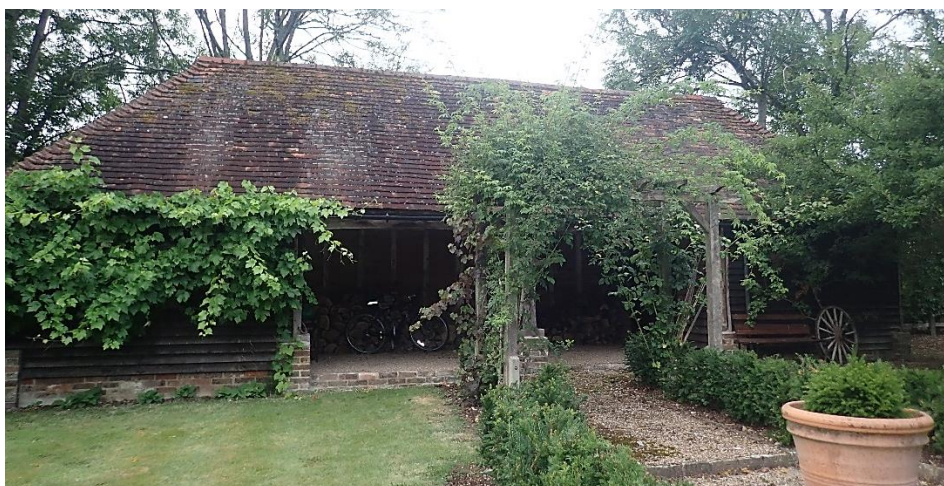
Fig. 2 – The barn, viewed from the south-east
