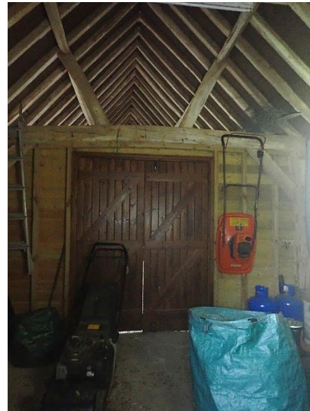
Fig. 4 – Partially enclosed room, N end (July 2025)
