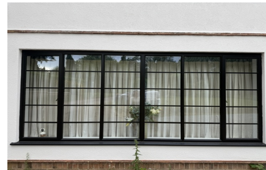
Existing Crittall-style lounge window
