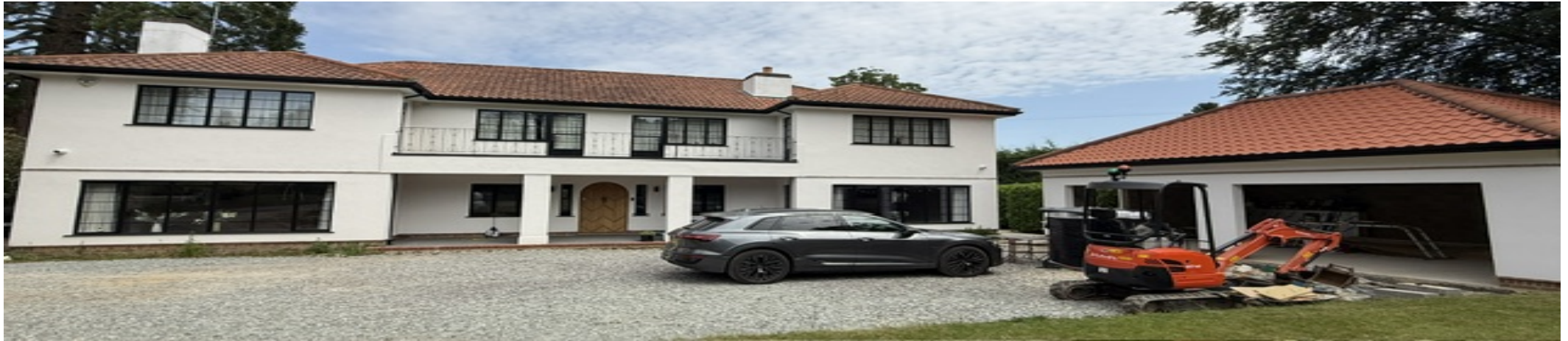
Finished house and garage under construction
