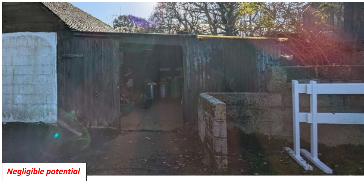
Figure 16. Preliminary Roost Assessment of B6 on site (taken November 2024, facing south)
