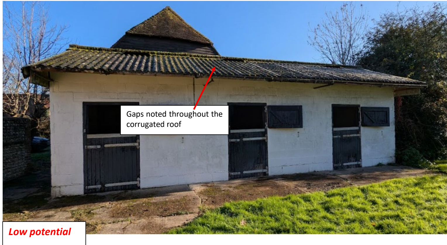
Figure 13. Preliminary Roost Assessment of B3 on site (taken November 2024, facing east)
