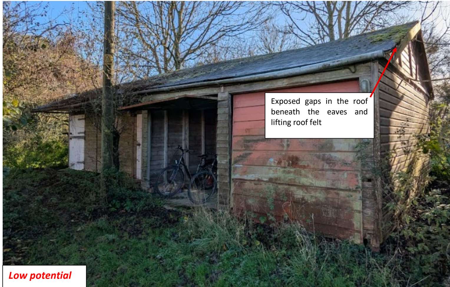
Figure 15. Preliminary Roost Assessment of B5 on site (taken November 2024, facing southeast)
