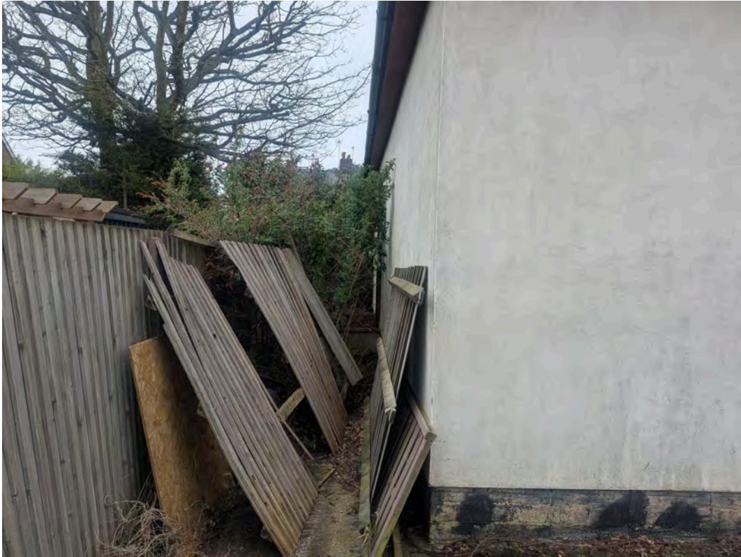
Photo 5: View of the southern boundary.
