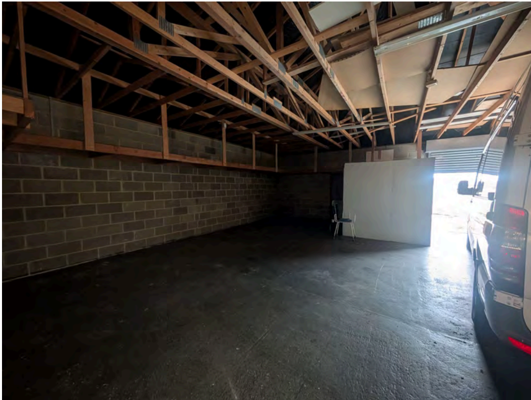
Photo 9: View of the north of the warehouse and office area.
