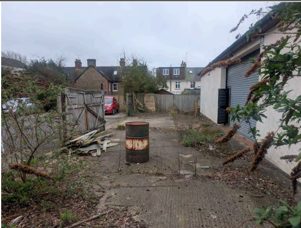
Photo 4: View of the external area of the Site from the north looking south.
