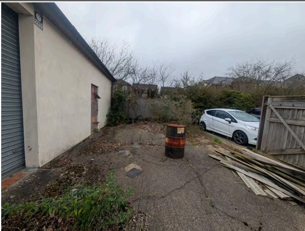
Photo 2: View of the external area of the Site from the centre looking north.
