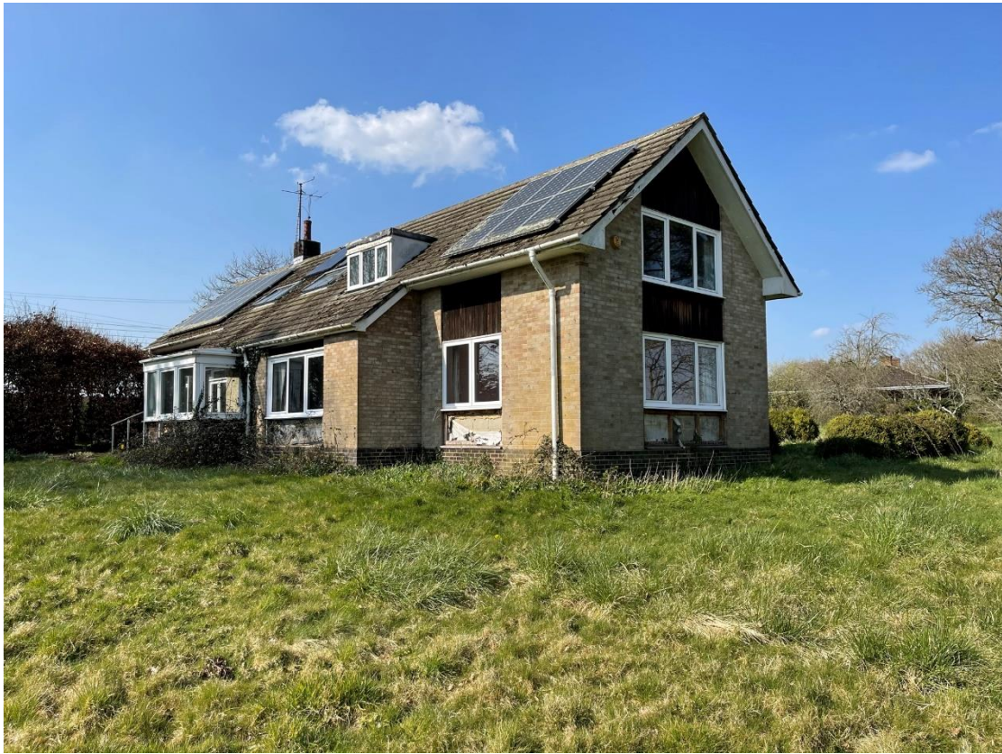
Image 01 – Showing the existing East Hookers Dwelling
