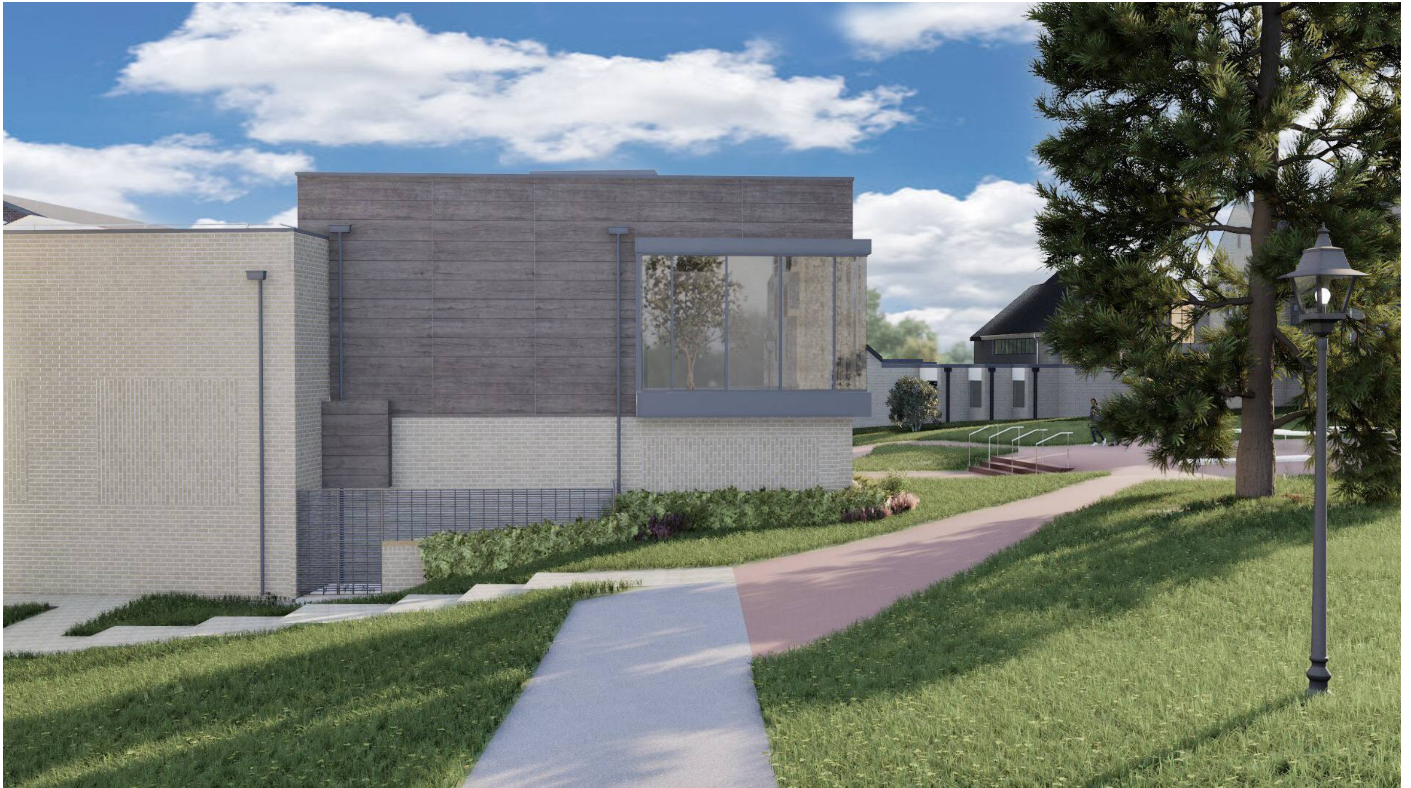
3.9 Exterior view of the building from the eastern (carpark) approach to the Quad .
