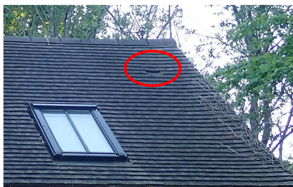
Fig. 4 – Missing roof tile on E facing roof slope, The Coach House
