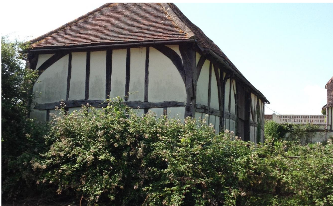
Photo of existing East Elevation
