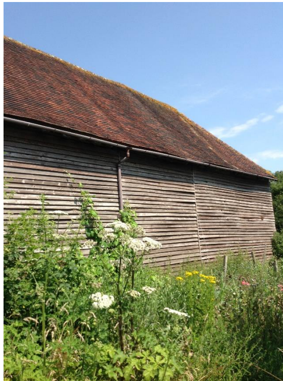
Photo of existing South Elevation
