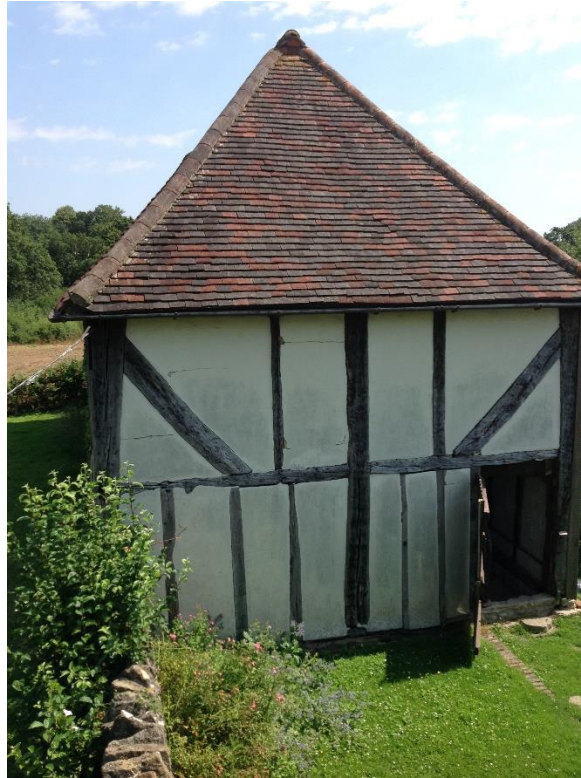
Photo of part of the existing West Elevation
