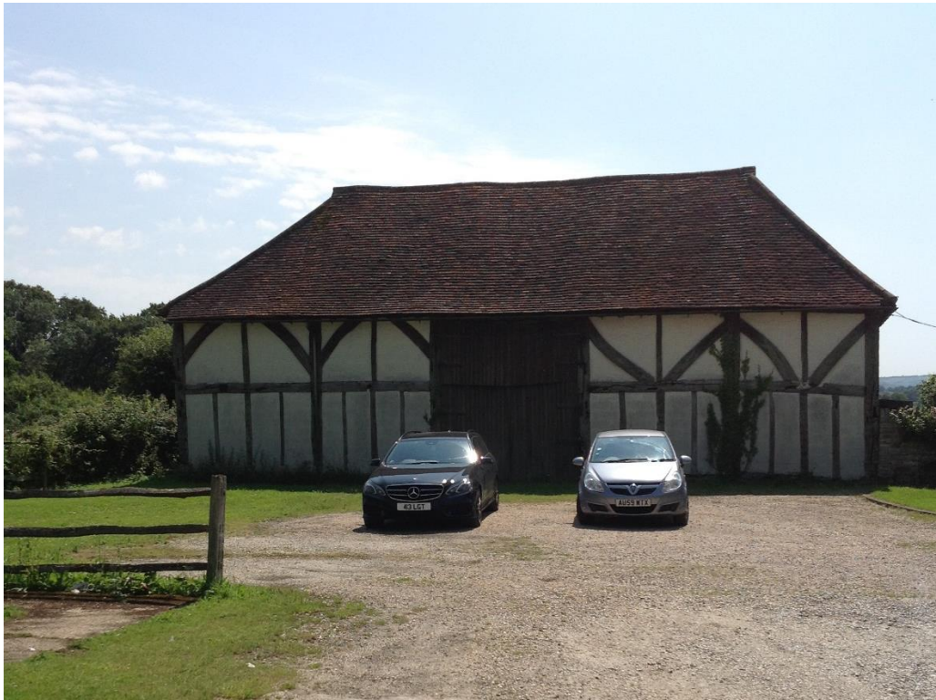
Photo of existing North Elevation
