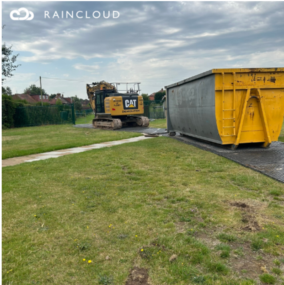
Figure 4: Typical Track Matting
