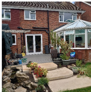
3 steps have been introduced to reduce from deck level to sunken garden level
